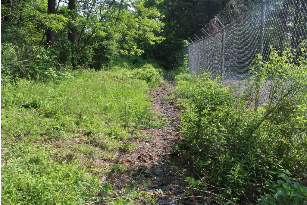
Photograph 9: General view of Basin 1095, located adjacent to Tanite Road west of US 209, facing northeast. The majority of the basin extent is located within the adjacent parking lot. Disturbed soil profiles were likely associated with the construction of the adjacent medical facility and parking lot.
