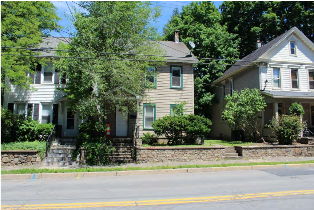
Photograph 85: General view of 36MR0282, facing east.
