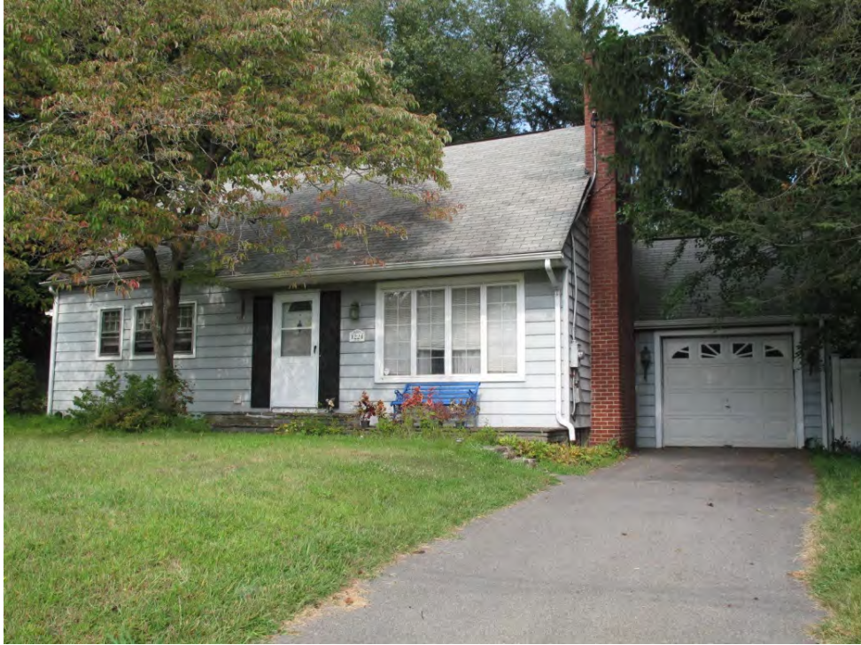
Photograph 60: General view of 36MR0255, facing west.
