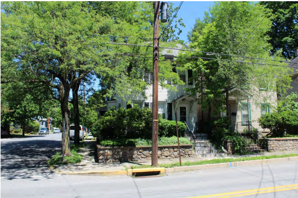
Photograph 83: General view of 36MR0252, facing east.
