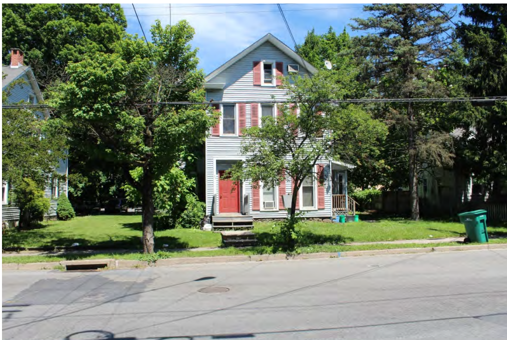
Photograph 78: General view of 36MR0278, facing east.
