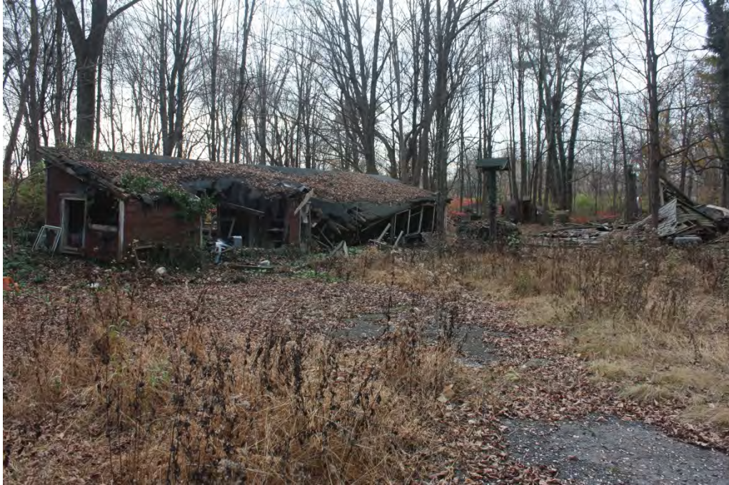
Photograph 47: General view of outbuildings at 36MR0283, facing southwest. Note shed and well in foreground and stone foundation for additional shed in background.
