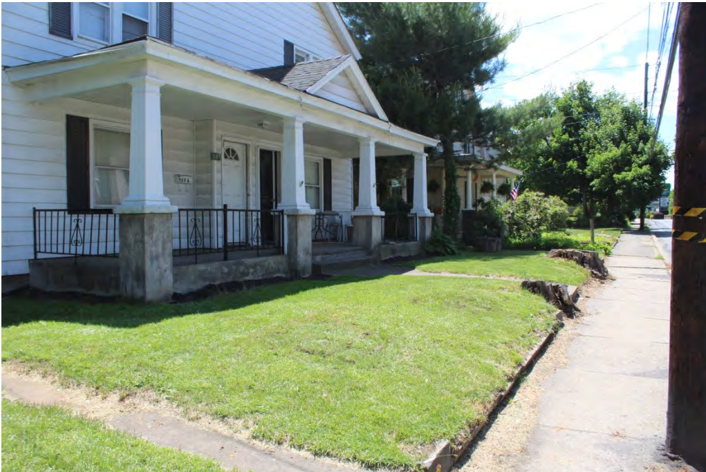
Photograph 38: General view of 36MR0262, facing west.
