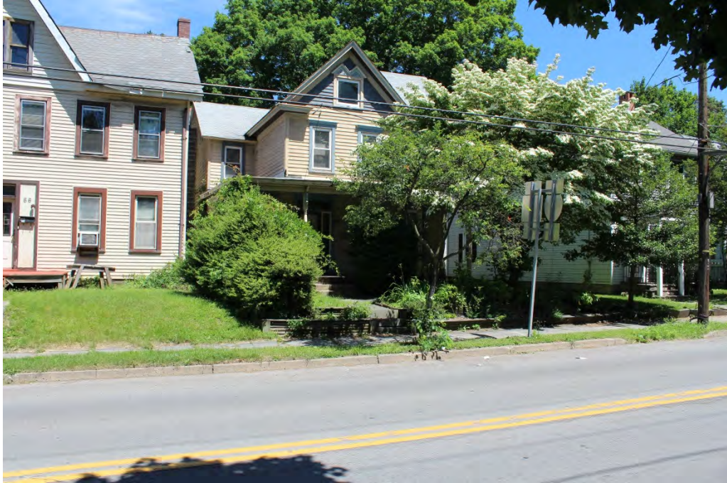
Photograph 80: General view of 36MR0249, facing east.
