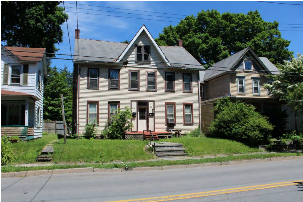
Photograph 81: General view of 36MR0250, facing east.
