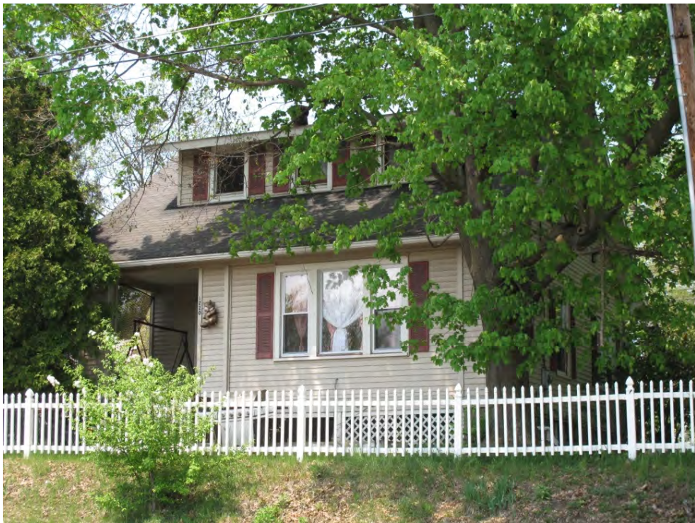
Photograph 61: General view of 36MR0273, facing west.
