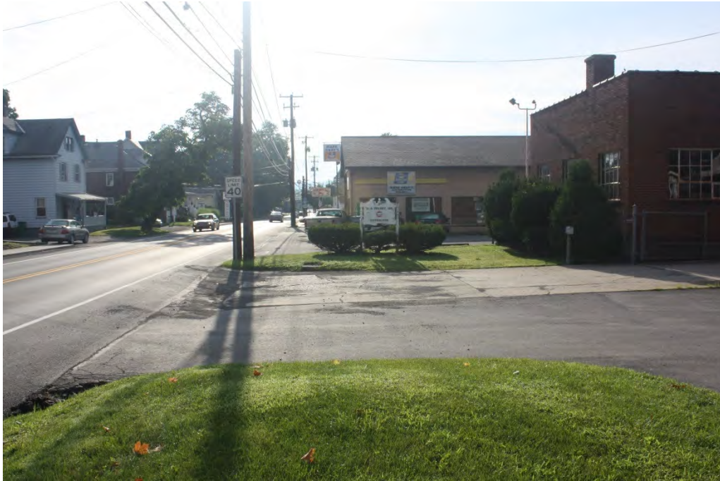
Photograph 29: General view of disturbance (graded and paved areas) as well as tested areas along W. Main St., between U.S. 209 and I-80, facing east.
