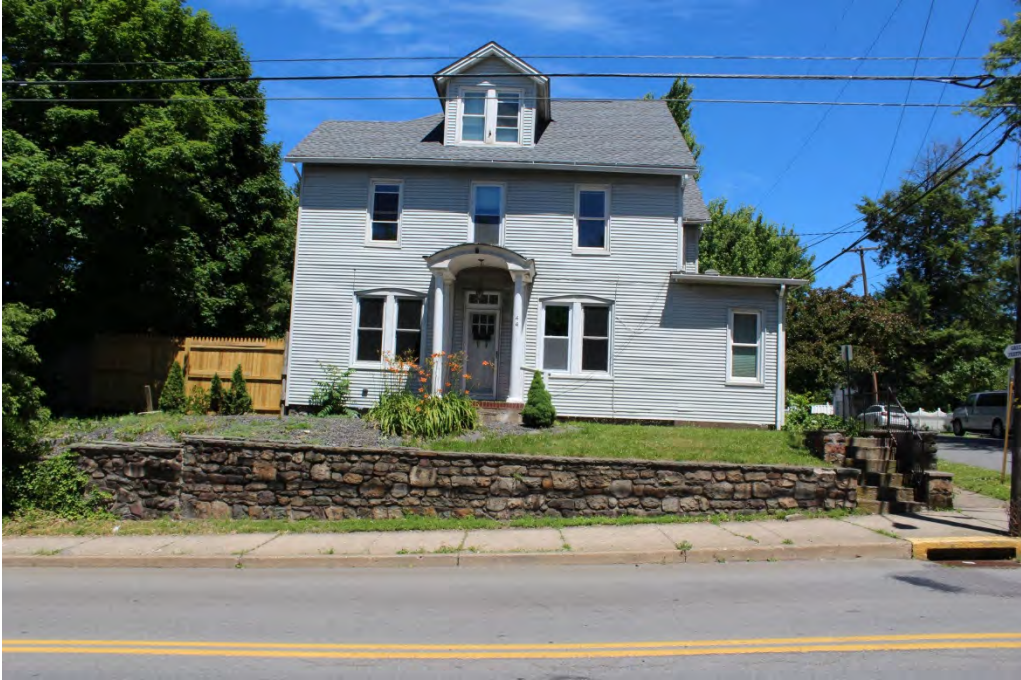
Photograph 84: General view of 36MR0253, facing east.
