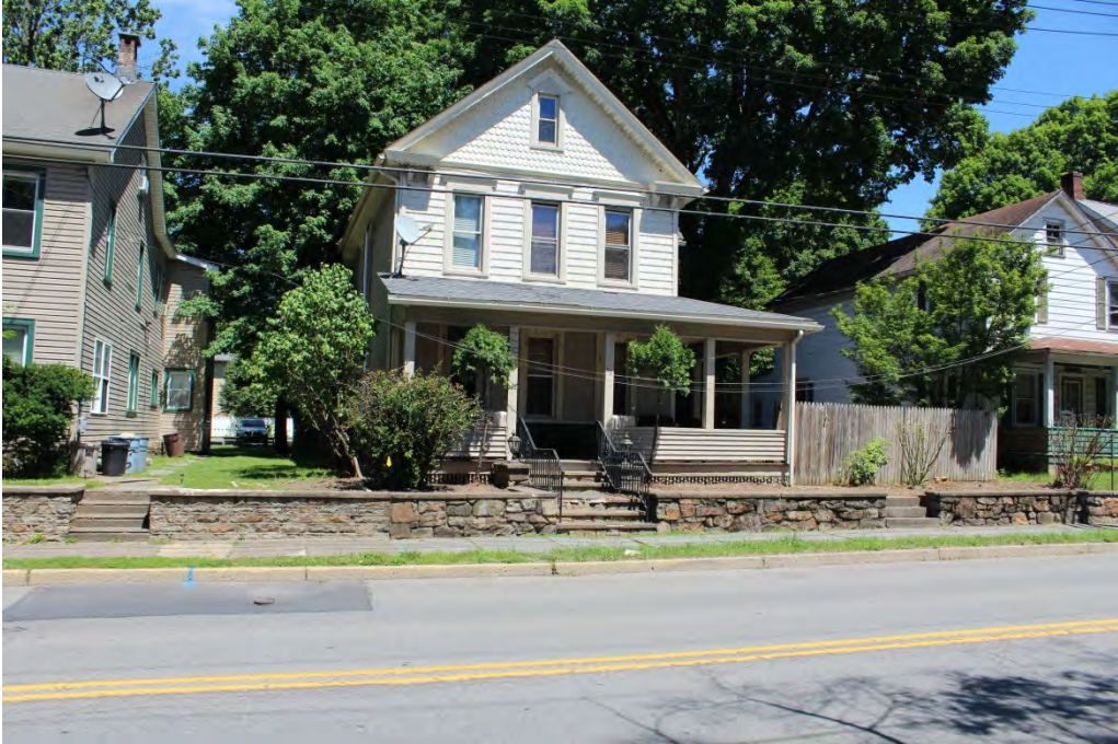
Photograph 82: General view of 36MR0251, facing east. Note demarcated buried utility.
