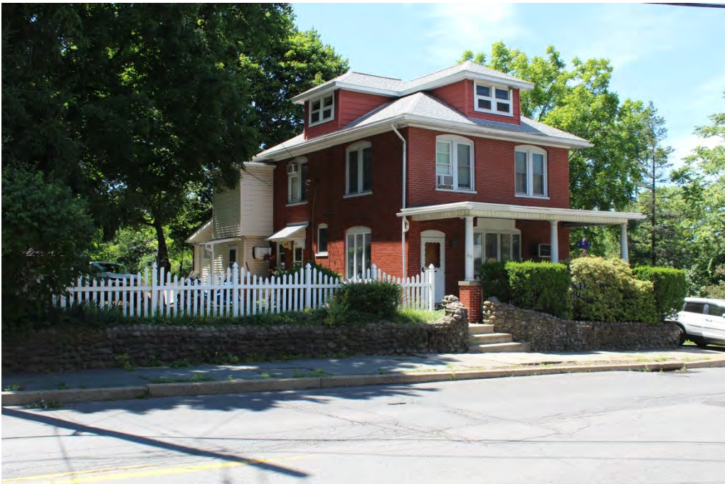
Photograph 73: General view of 36MR0275, facing northwest.
