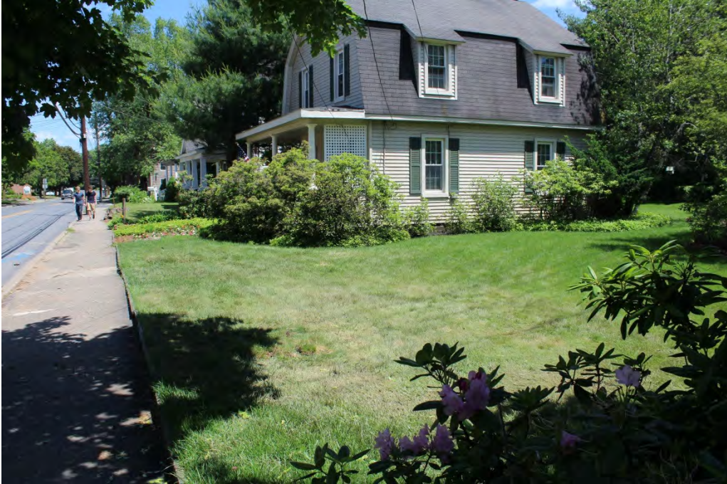
Photograph 37: General view of 36MR0261, facing east.
