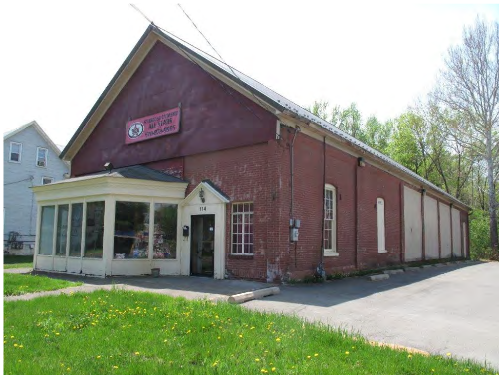
Photograph 69: General view of early twentieth century Stroudsburg & Water Gap Street Railway trolley barn (Key# 038810) associated with 36MR0248, facing west.
