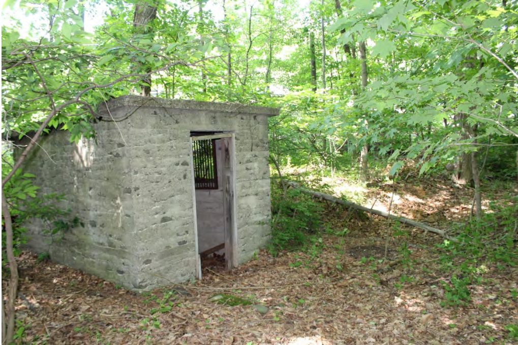
Photograph 115: General view of springhouse (Feature 15) and associated waste water holding pond (Feature 16) at 36MR0283, facing east. Note location of STP 184 at right.
