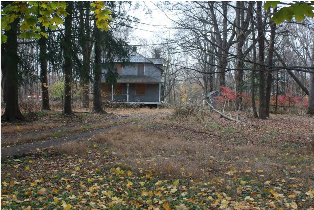
Photograph 46: General view of residence at 36MR0283, facing west.
