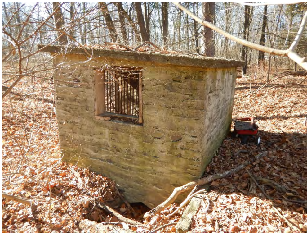
Photograph 48: General view of springhouse at 36MR0283, facing west.
