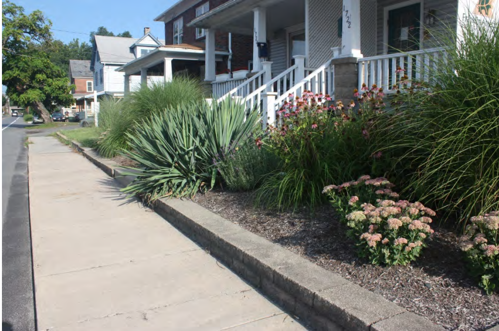
Photograph 33: General view of 36MR0269, facing west.
