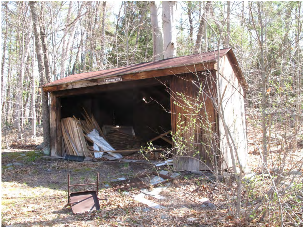
Photograph 6: View looking northeast at the Kirkwood Shed.
