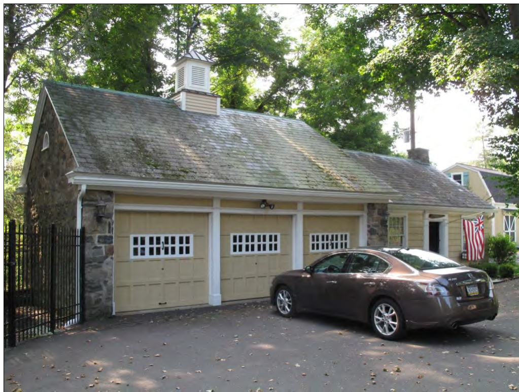
Photograph 7: View looking south at the garage/work shop.
