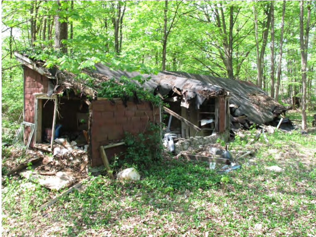
Photograph 7: View looking southwest at the Chicken House/Storage Shed.
