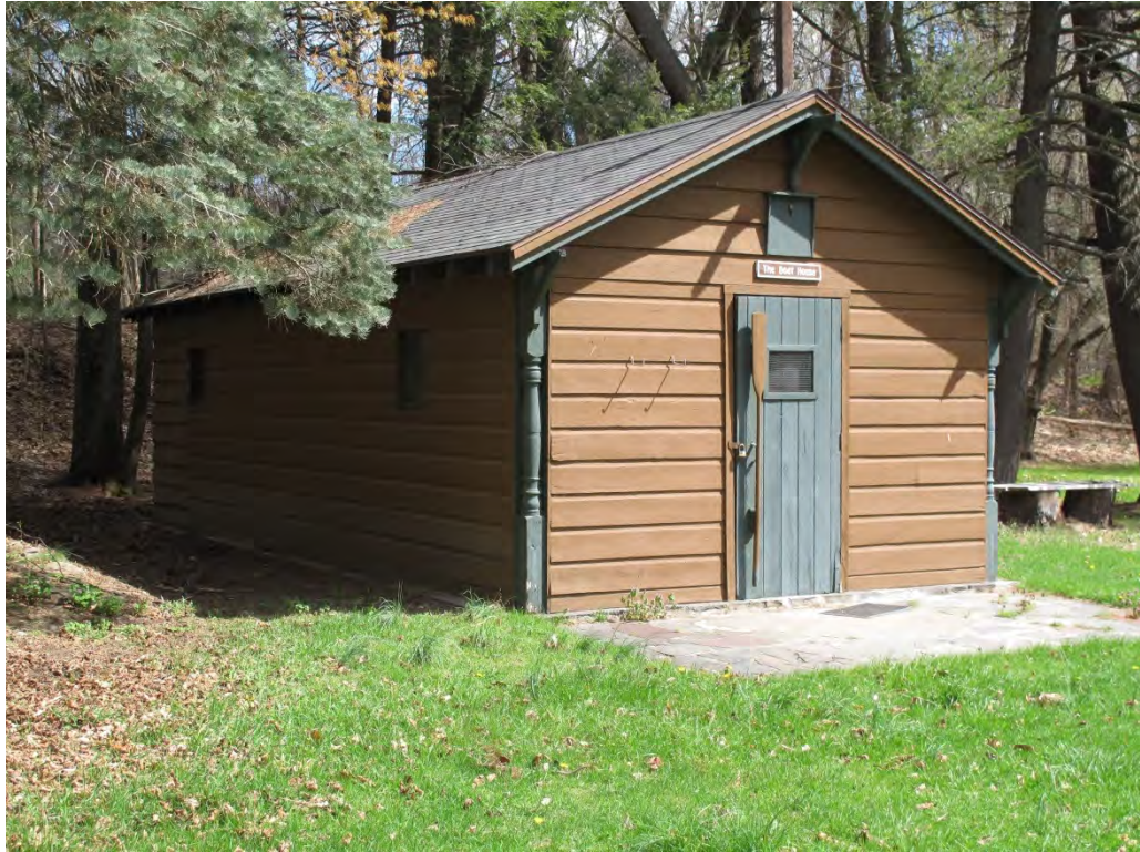
Photograph 23: View looking northeast at the Boat House.
