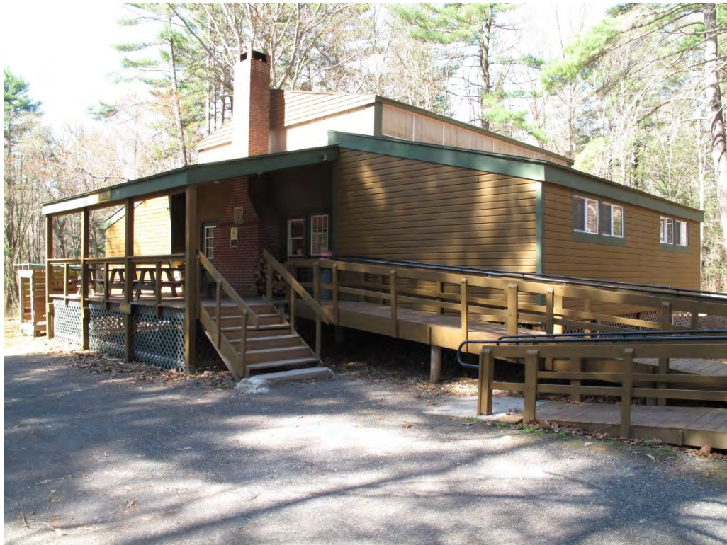
Photograph 10: North and east elevations of the Stroup House.
