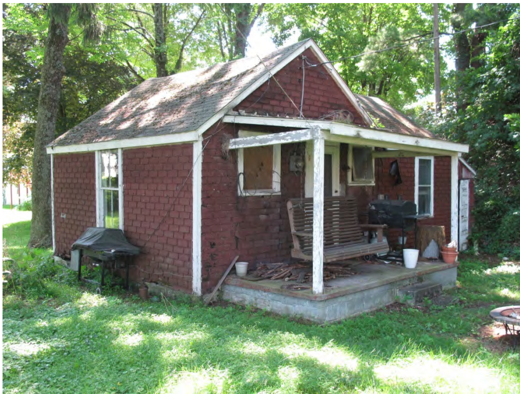
Photograph 5: North and west elevations of the cottage.
