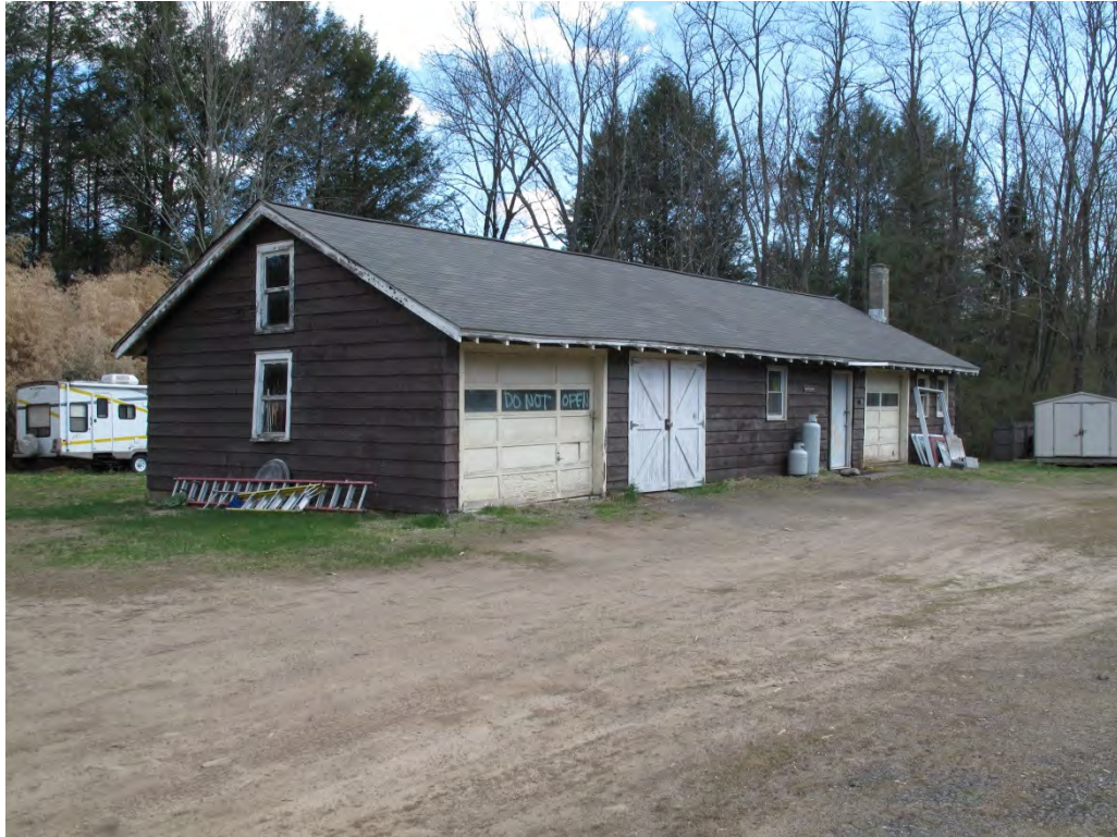
Photograph 17: West and south elevations of the Pony Barn.
