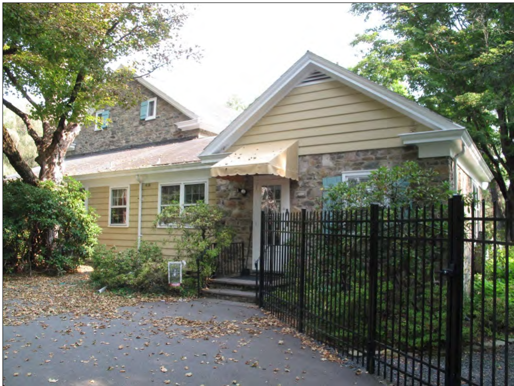
Photograph 6: View looking northeast at the west elevation of the Stroud-Hollinshead House, showing a twentieth century addition connected to the stone summer kitchen.
