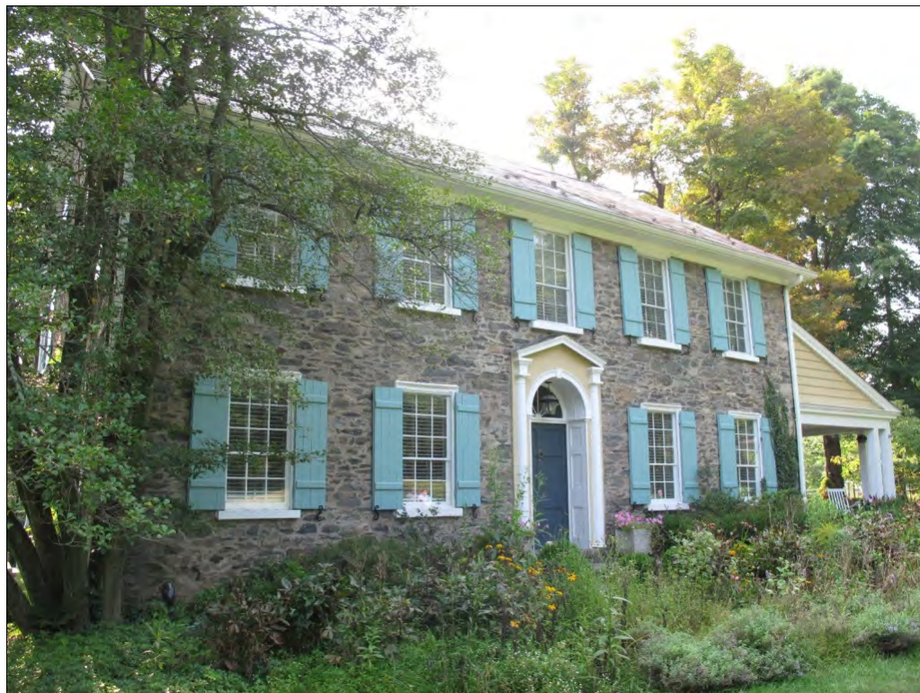
Photograph 3: View looking southwest at the façade of the Stroud-Hollinshead House.
