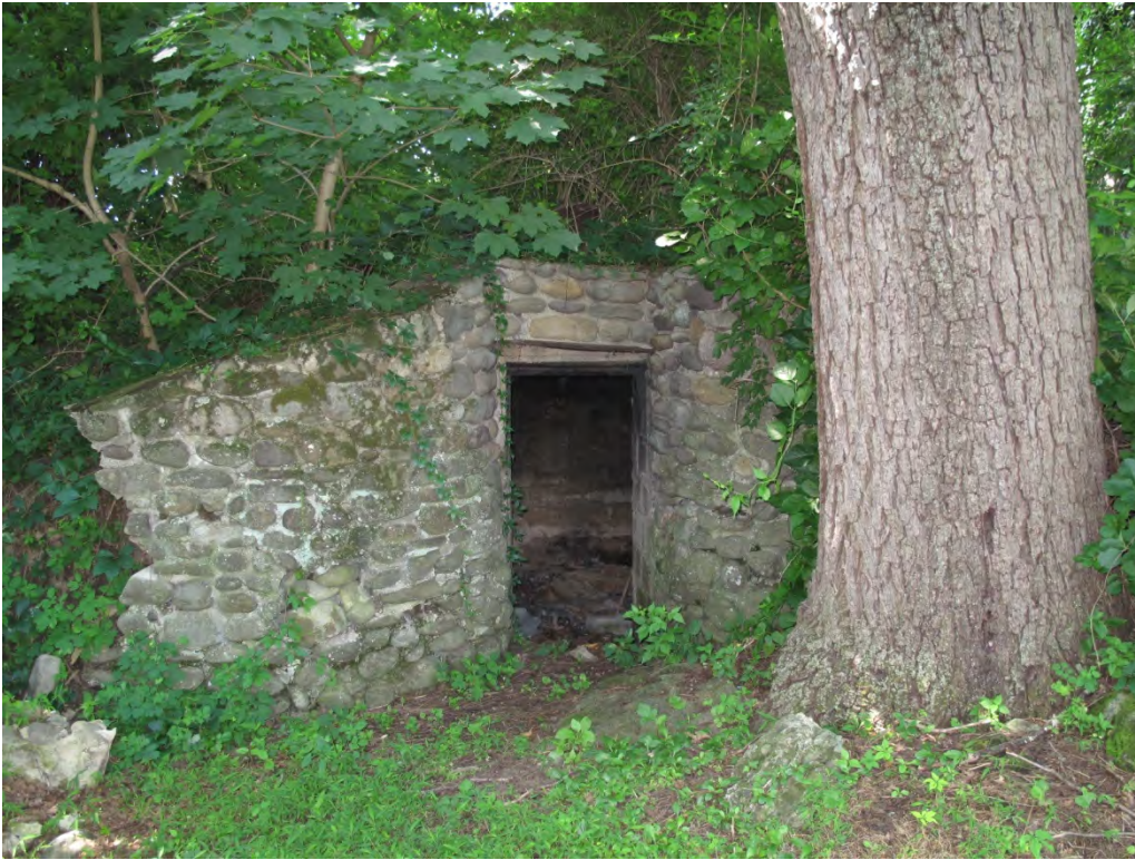
Photograph 7: View looking south at the stone cellar.
