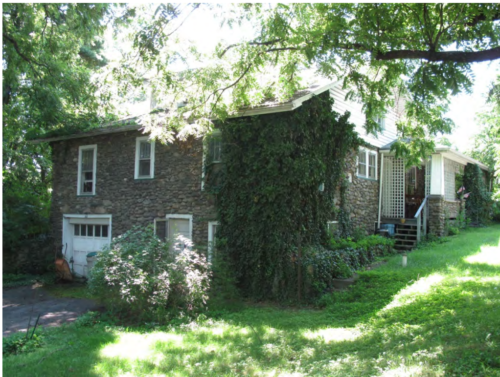
Photograph 3: West and north elevations of the Mengle House.
