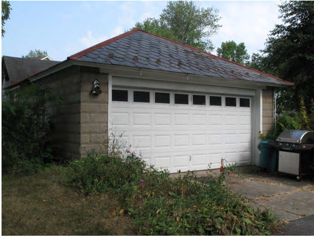
Photograph 7: South and east elevations of the concrete block garage.
