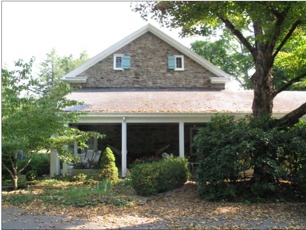
Photograph 5: View of west elevation of the Stroud-Hollinshead House, including porch addition.
