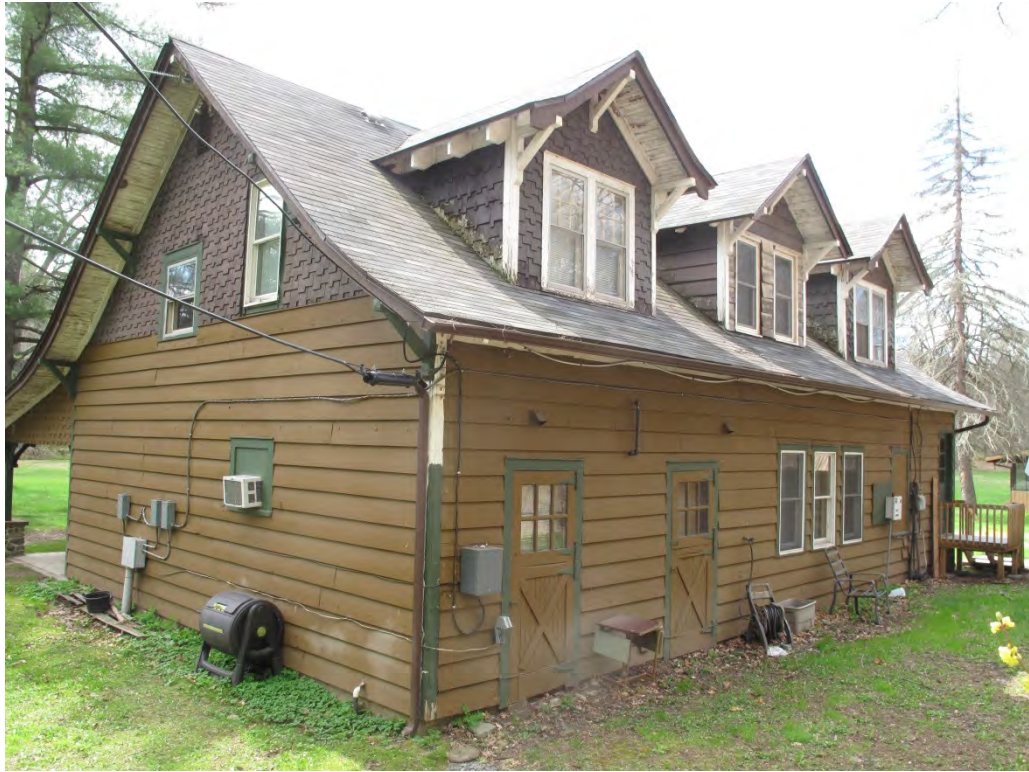
Photograph 25: View looking south at the Carriage House. Note the Craftsman style elements, including patterned shingles, exposed rafters and brackets.
