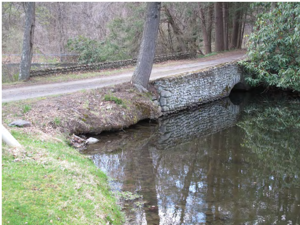
Photograph 22: View looking southeast at the Stone Bridge.
