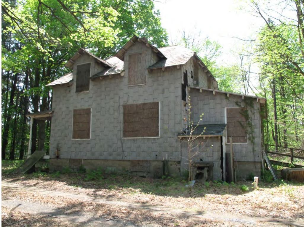
Photograph 3: View of the north elevation of the Palmer House.
