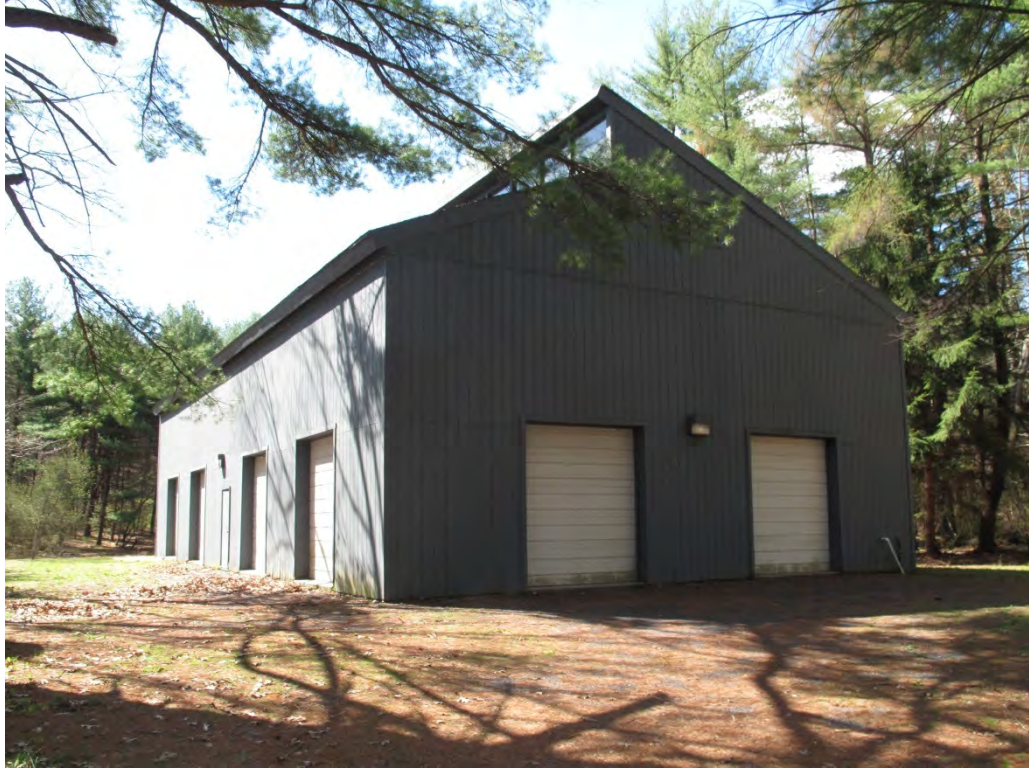
Photograph 15: South and east elevations of Bob's Depot (Maintenance Building).
