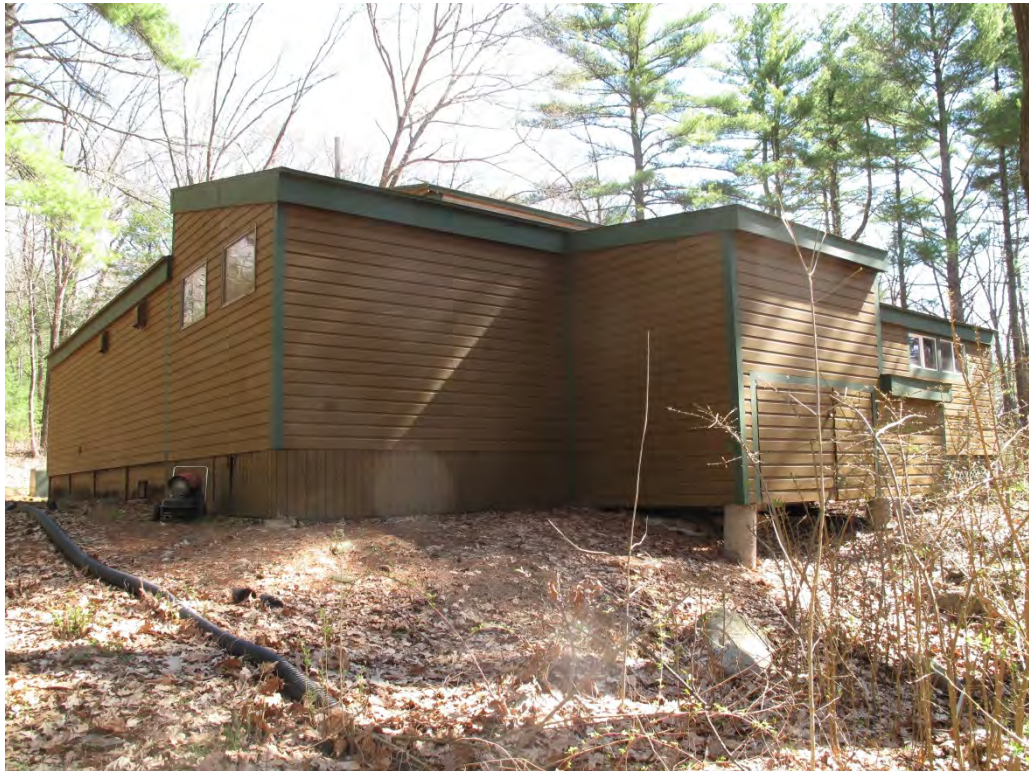
Photograph 11: South and west elevations of the Stroup House.
