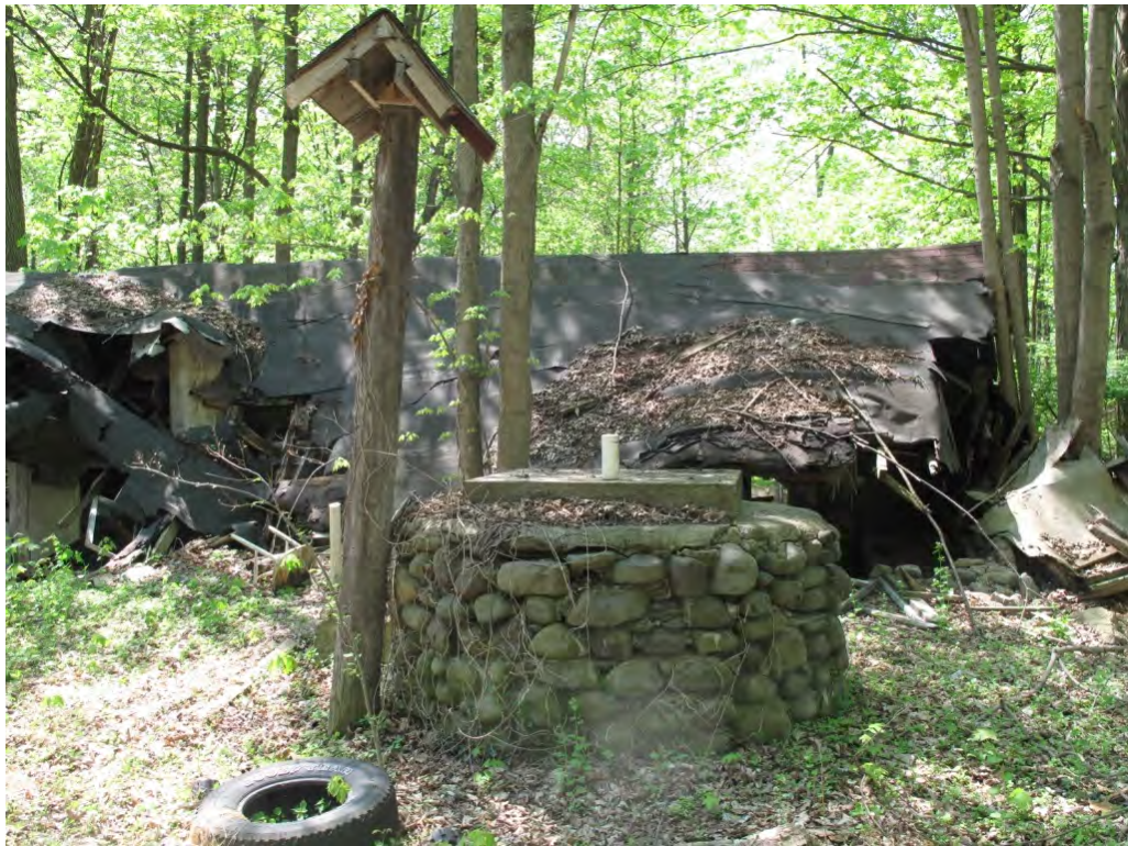
Photograph 6: View looking south at the circular, cobblestone well is located west of the house.
