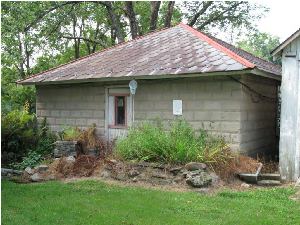
Photograph 8: North and west elevations of the concrete block garage.
