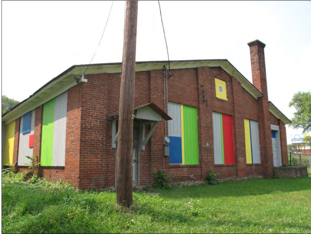
Photograph 1: North and east elevations of the former Perfection Shoe Machinery Company.
