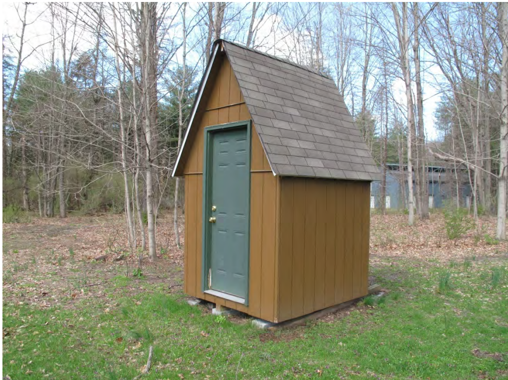
Photograph 16: View looking northwest at a modern utility shed.
