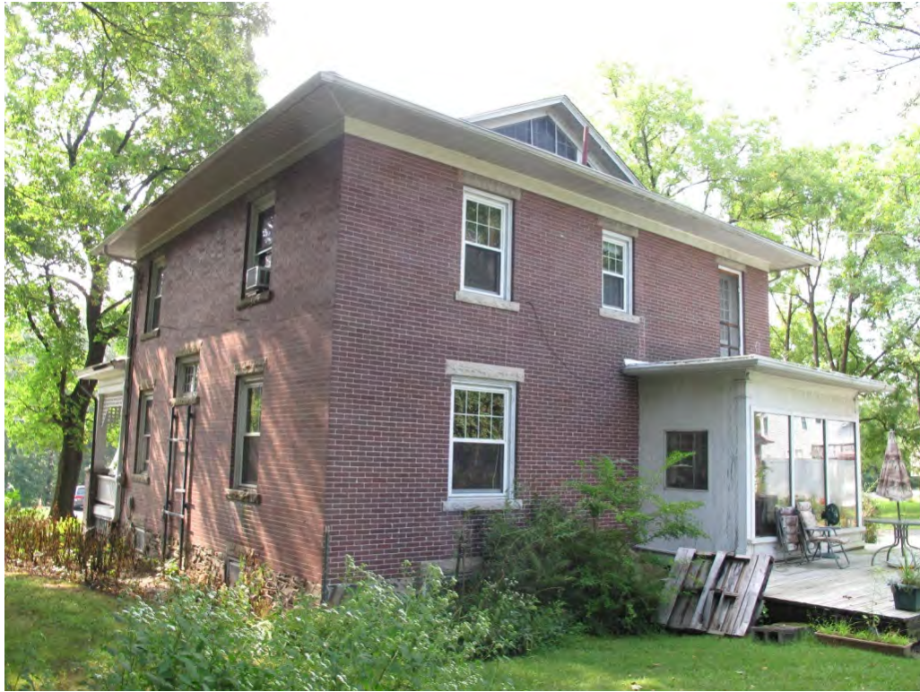
Photograph 5: North and East elevations of the Kautz-Kintz House.
