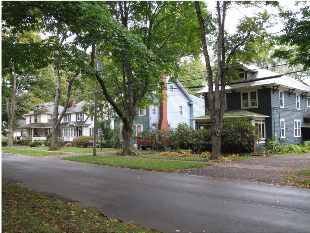
Photograph 19: View looking northwest at residences located along the north side of Bryant Street.
