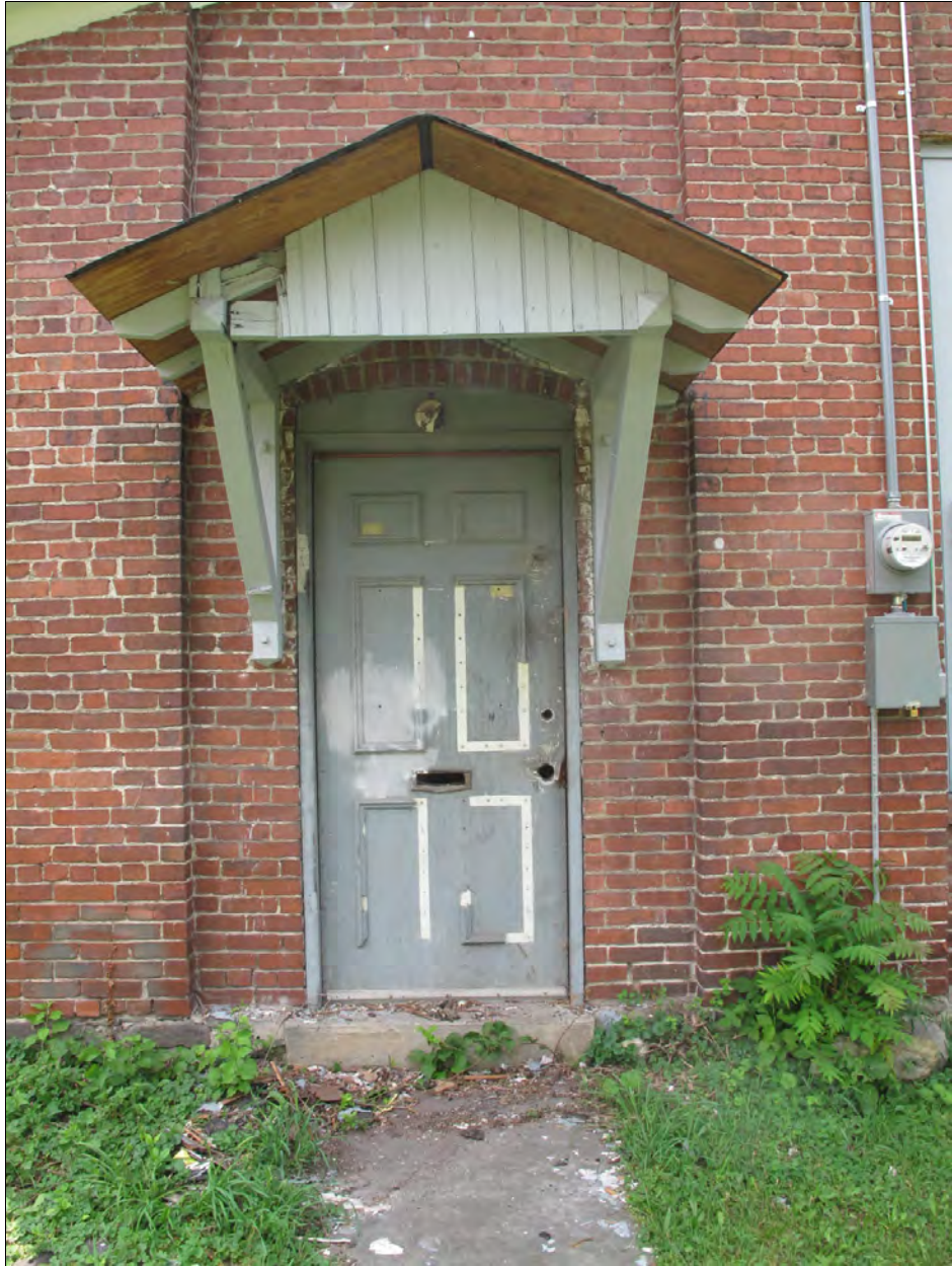
Photograph 3: Detail of main entrance located at northeast corner of the building.
