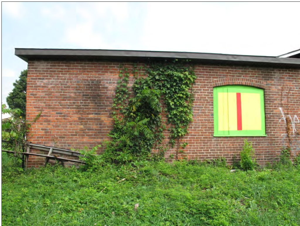
Photograph 7: South elevation of the one-story wing addition.
