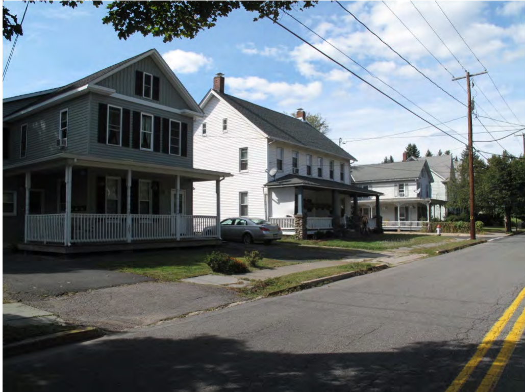
Photograph 2: View looking northwest along Broad Street from Robeson Street.
