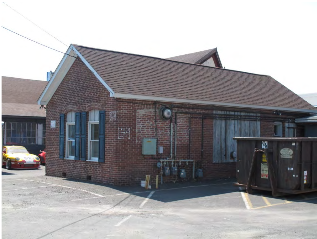
Photograph 1: View looking southeast at the north and west elevations of the office building section of the former H.B. Marsh & Son, Inc. foundry.
