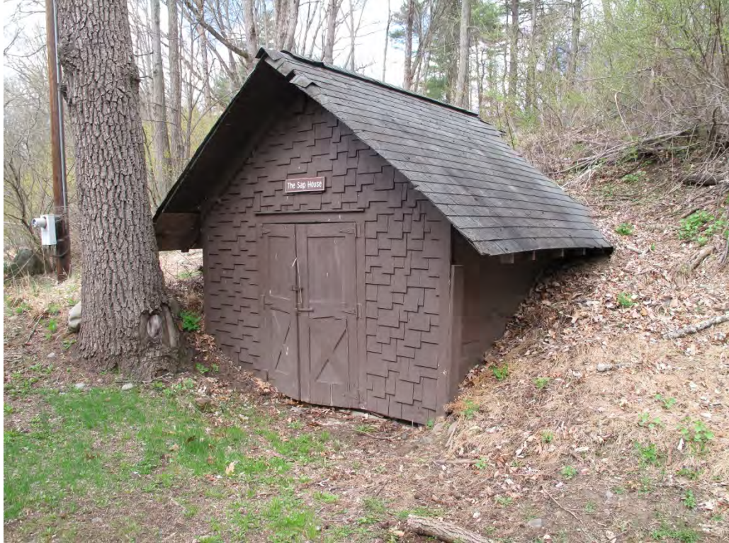
Photograph 26: View looking north at the Sap House.
