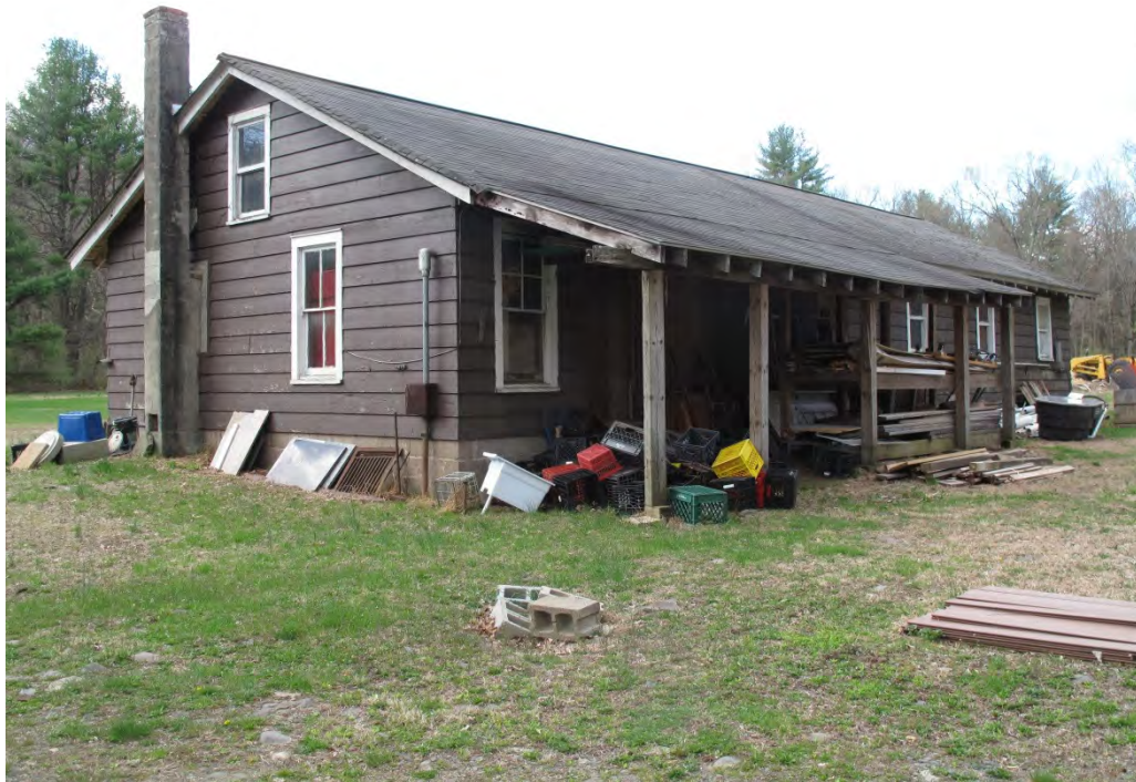
Photograph 18: North and east elevations of the Pony Barn.
