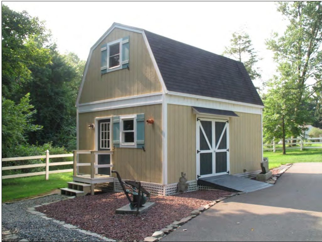
Photograph 9: View looking southwest at the modern gambrel roof shed.
