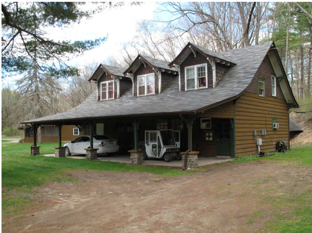
Photograph 24: View looking at the south and east elevations of the Carriage House.
