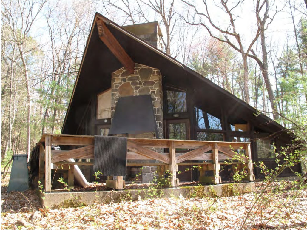
Photograph 7: View looking northwest at 312 Kirkwood Road.
