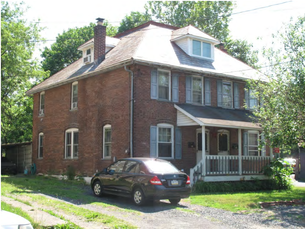
Photograph 10: View looking east at the north and west facing façade of the house at 10/12 Foundry Street.
