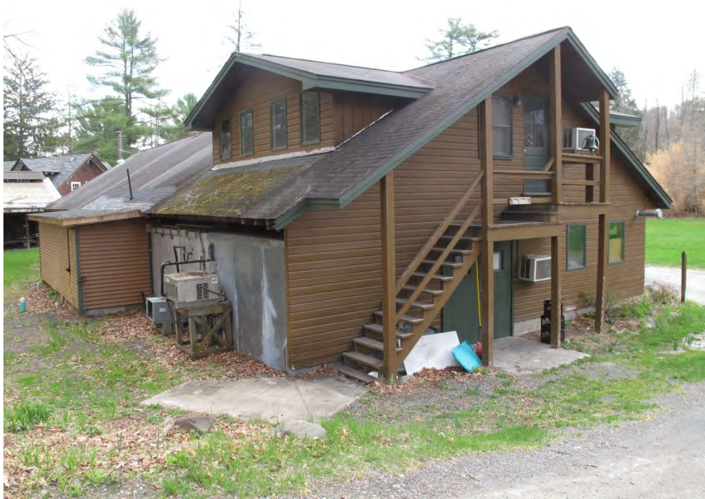
Photograph 29: North and west elevations of The Coop.
