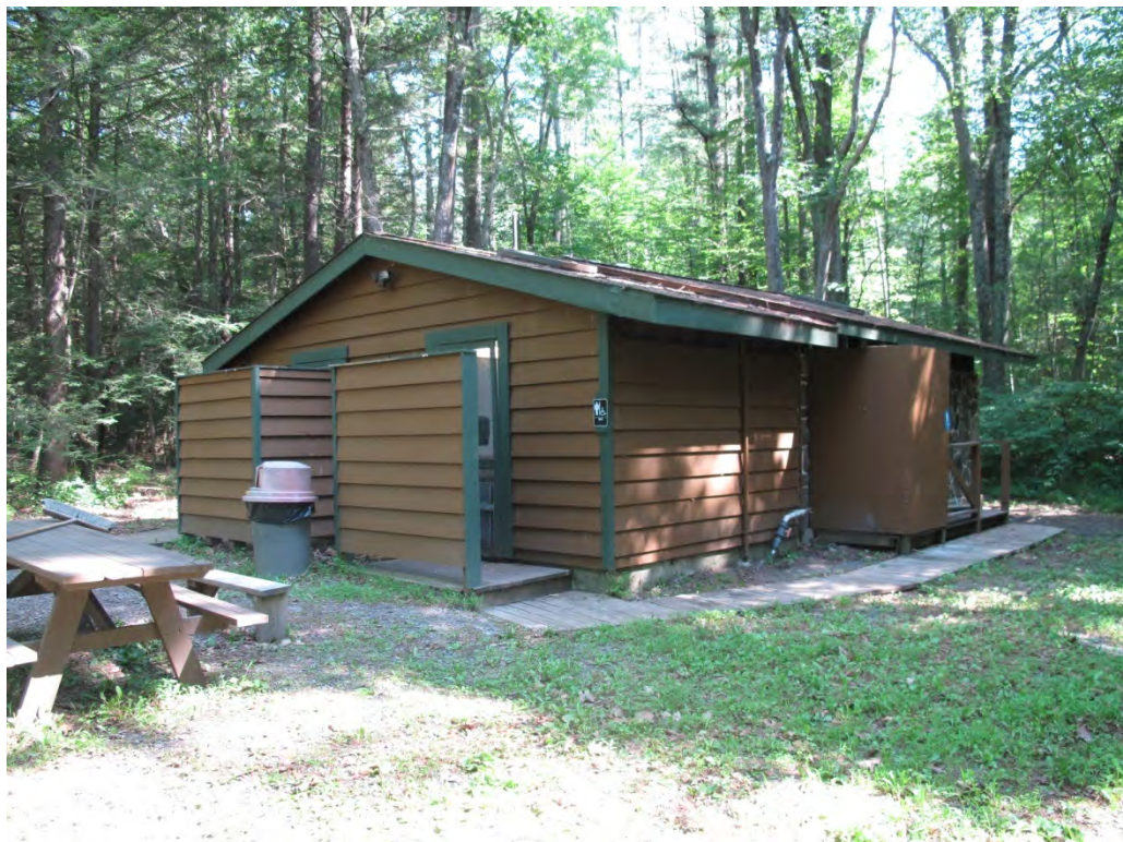
Photograph 12: View looking northwest at the Bath House.
