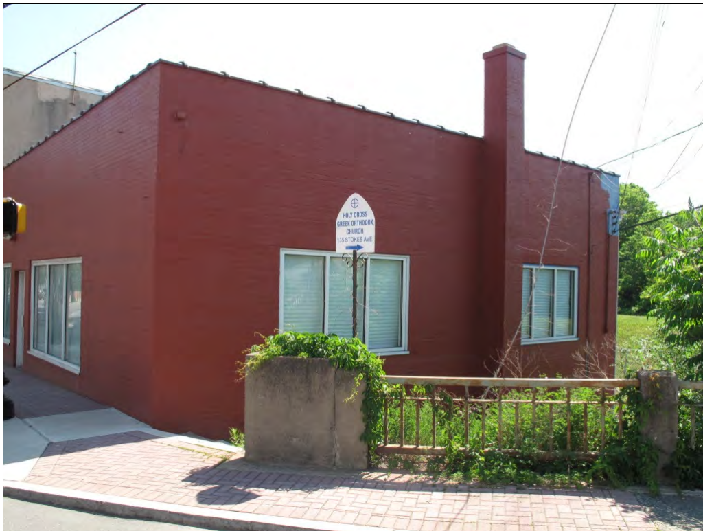
Photograph 2: West and north elevations of the Stroudsburg Motor Supply Company building.
