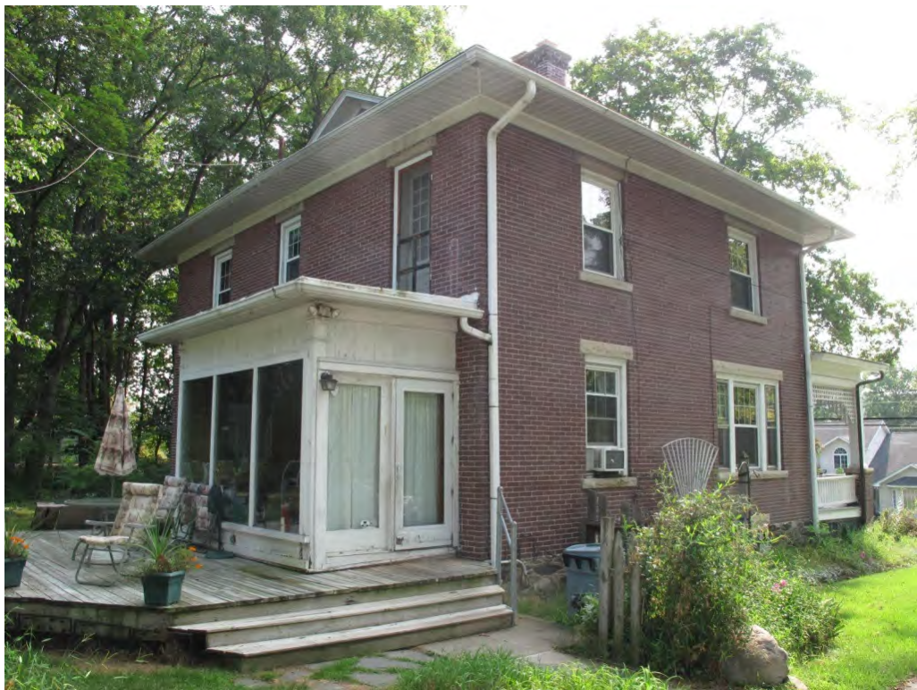
Photograph 6: South and west elevations of the c. 1915 Kautz-Kintz House.
