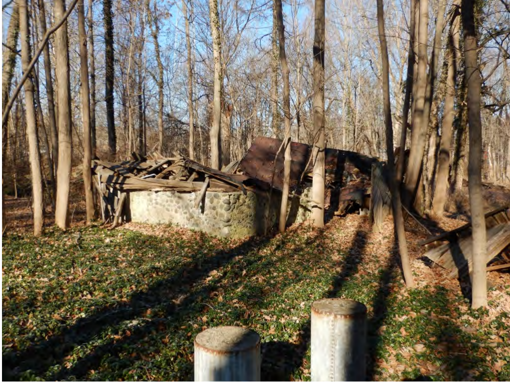
Photograph 9: View of the storage shed ruins.
