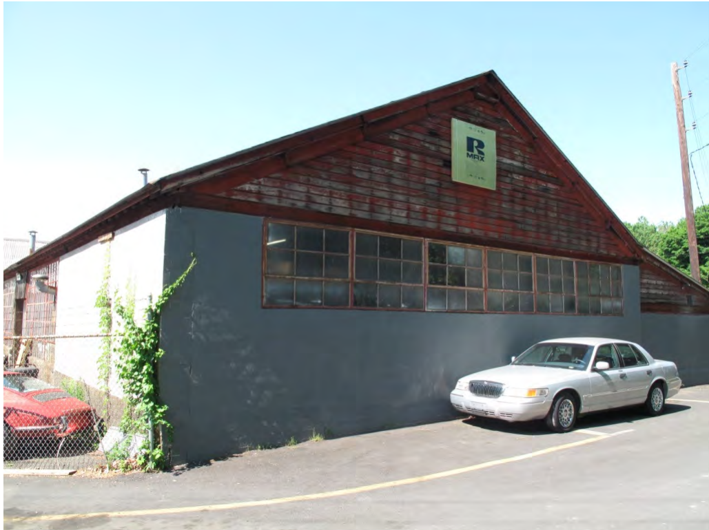
Photograph 5: View looking southwest at the north and east elevations former H. B. Marsh & Son, Inc. foundry.
