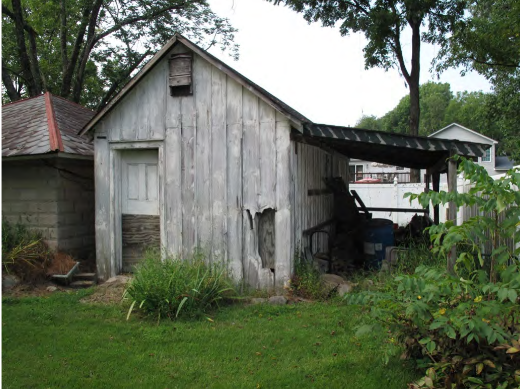
Photograph 9: View looking south at the frame wood shed, adjacent to the garage.
