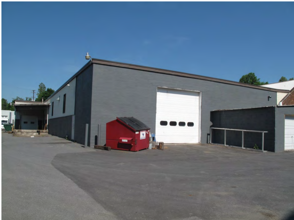
Photograph 6: View looking northwest at the east and south elevations of the former H. B. Marsh & Son, Inc. foundry.
