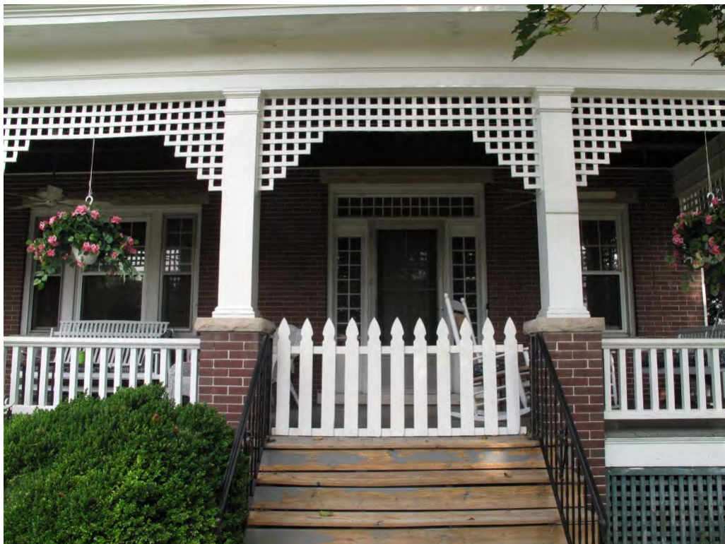
Photograph 4: View of porch and entrance of the Kautz-Kintz House.
