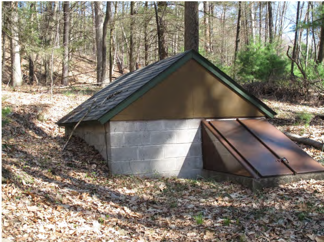
Photograph 8: View looking east at the concrete block springhouse.
