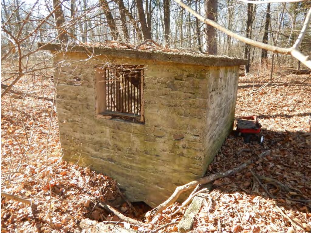
Photograph 11: View looking southwest at the spring house.
