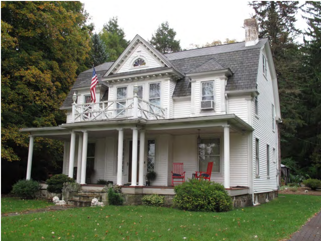
Photograph 28: North and west elevations of 50 Club Court.
