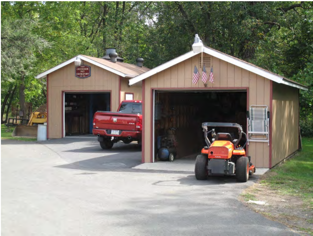
Photograph 9: View looking east at the west and north elevations of the Creekside Pet Crematory and a late twentieth century garage.
