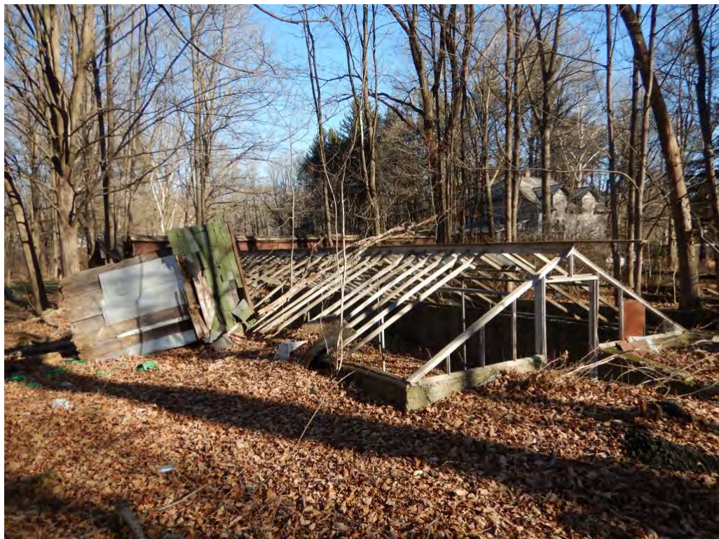
Photograph 8: View looking northeast at the greenhouse ruins.
