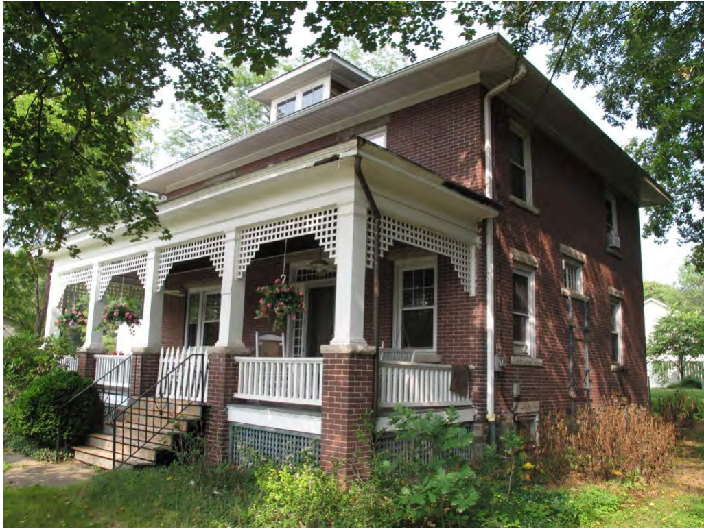
Photograph 3: North and east elevations of the ca. 1915 Kautz-Kintz House.
