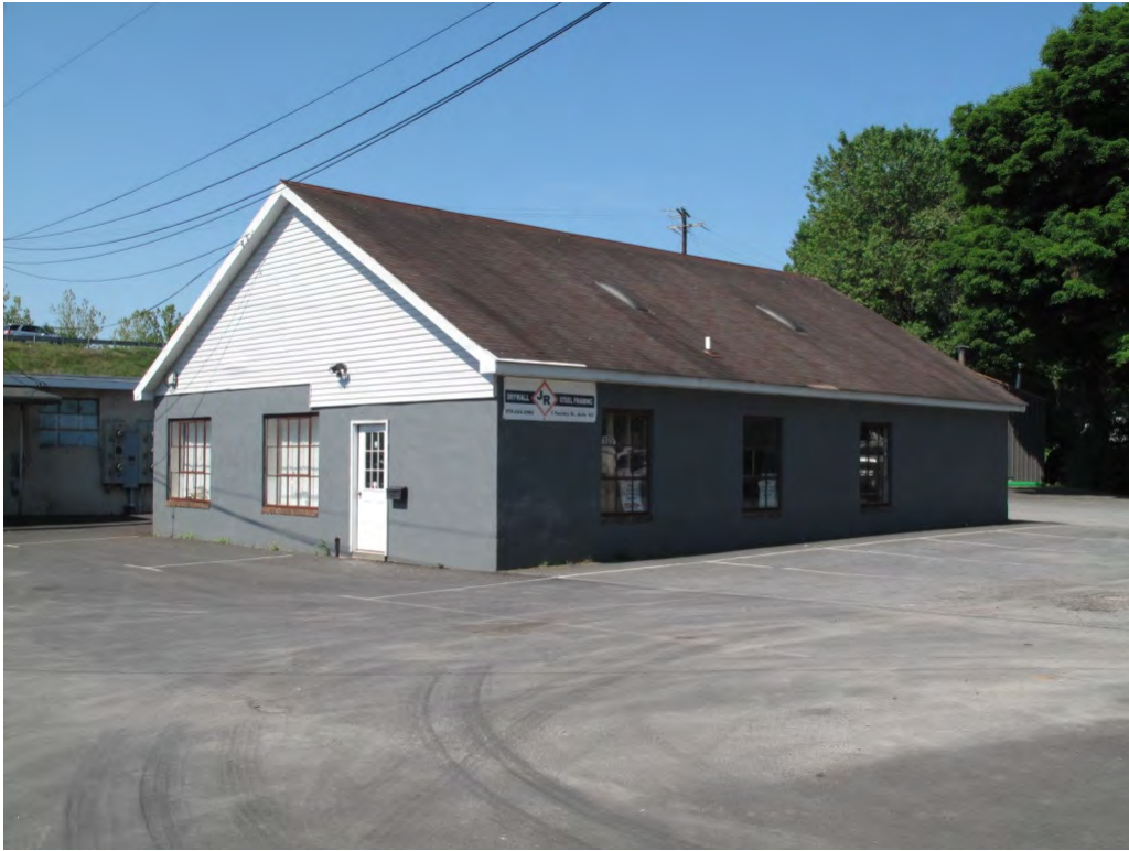
Photograph 9: View looking southwest at the north and east elevations of a building within the former H. B. Marsh & Son, Inc. foundry complex.
