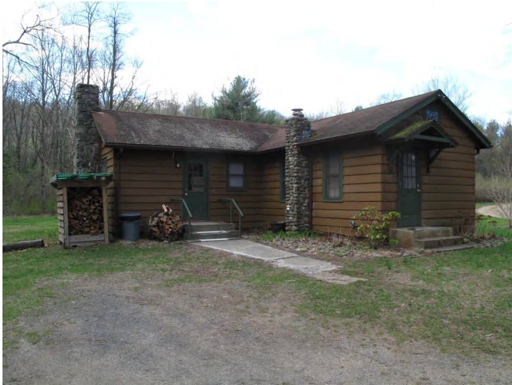
Photograph 21: North and east elevations of the Meadowside Cabin.
