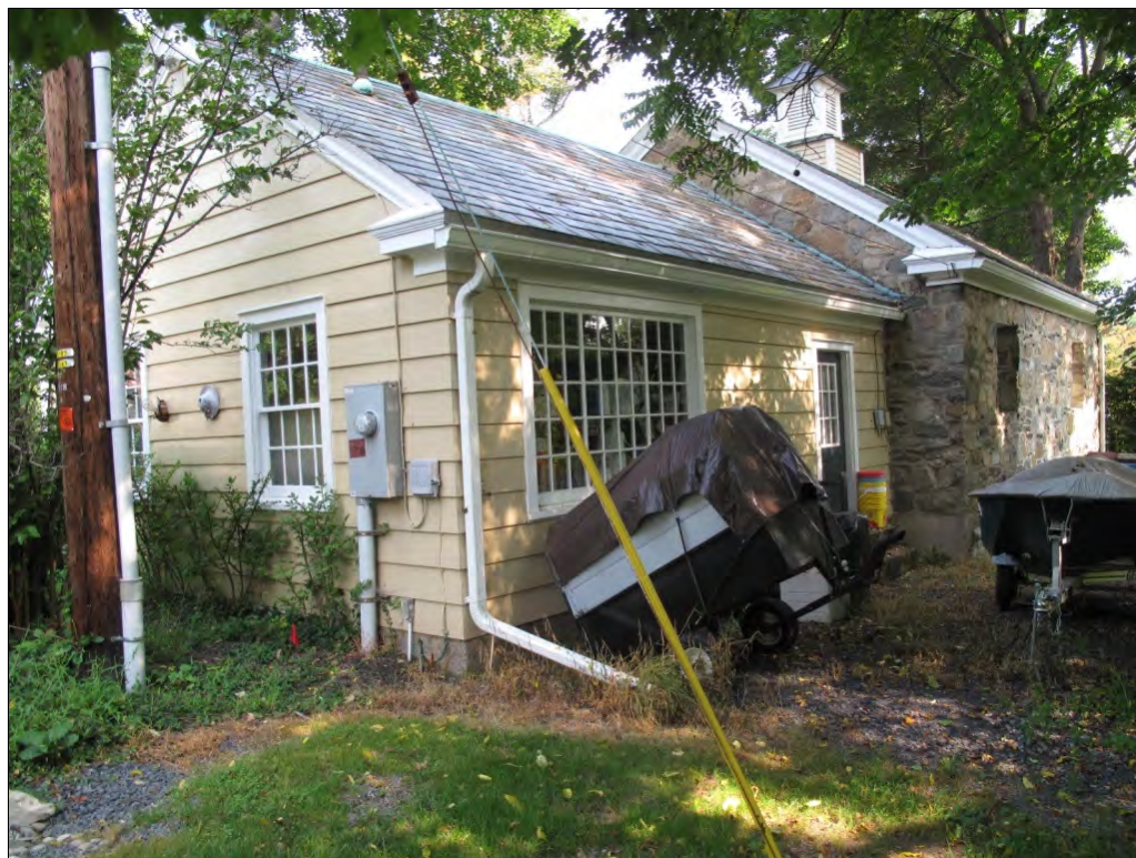
Photograph 8: View looking northeast at the rear of the garage/work shop.
