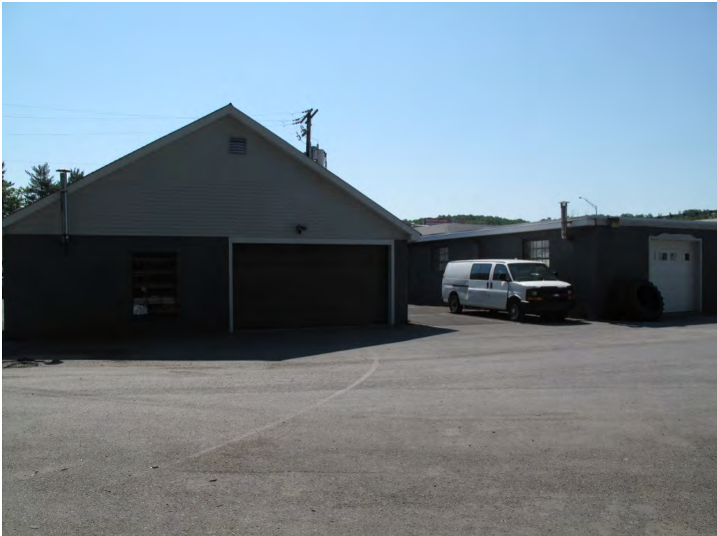
Photograph 8: View looking southeast at the north and west elevations of the former H. B. Marsh & Son, Inc. foundry.
