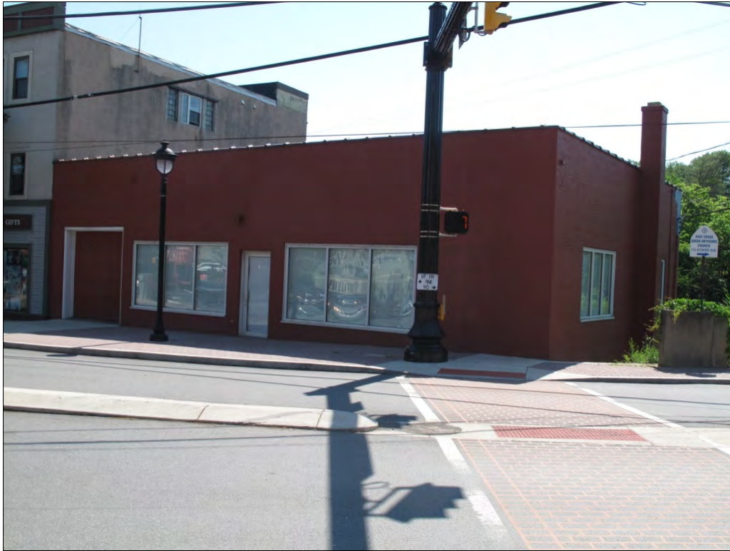
Photograph 1: North and west elevations of the Stroudsburg Motor Supply Company building.
