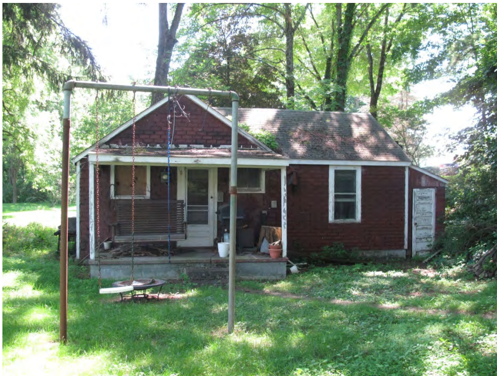
Photograph 6: West elevation of the cottage.
