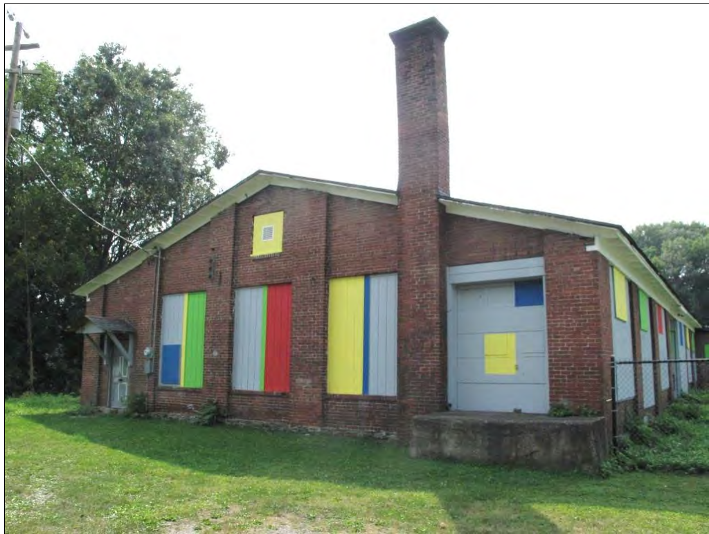
Photograph 2: North and west elevations of the former Perfection Shoe Machinery Company.
