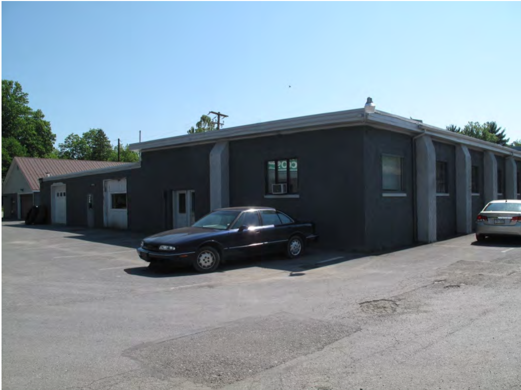
Photograph 7: View looking northeast at the west and south elevations of the former H. B. Marsh & Son, Inc. foundry.
