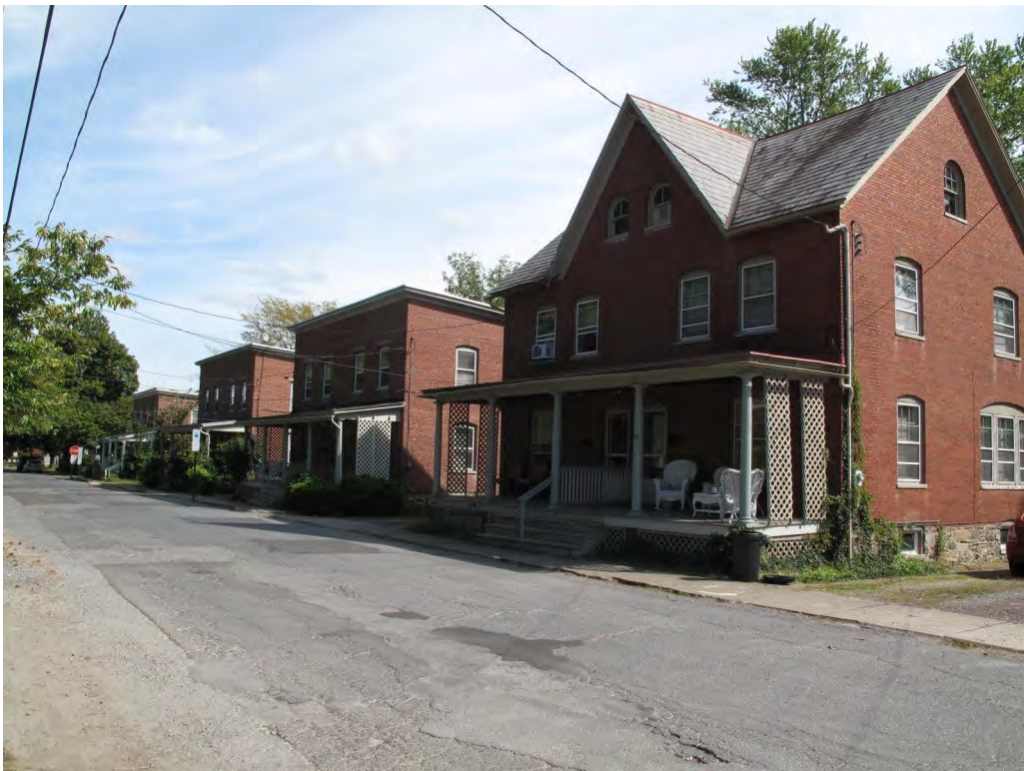
Photograph 12: View looking southeast along Collins Street.
