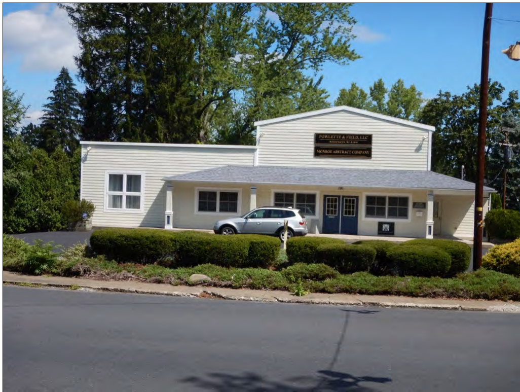
Photograph 32: Looking northeast from Morningside Avenue toward a modern office building along Park Avenue.
