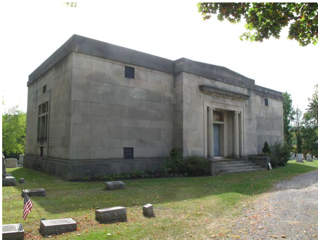
Photograph 6: View looking south at the north and east elevations of the Stroudsburg Memorial.
