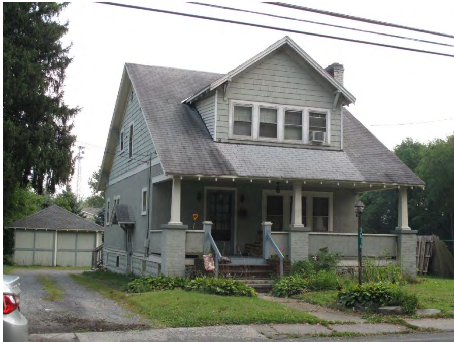
Photograph 4: View looking southeast at the west and north elevations of the house at 3616 Bridge Street.
