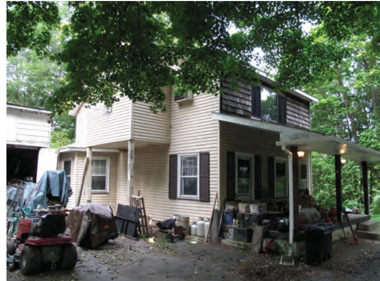
Caption: Photo 1: South and east elevations of 300 Tanite Road while facing north.
