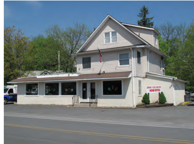
Caption: Photograph 1: View looking northwest at the south and east elevations of 1946 W. Main Street.
