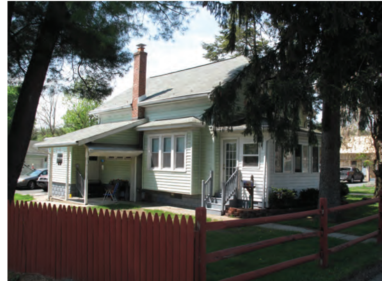
Caption: Photograph 1: Facade (right) and east elevation of 1933 West Main Street while facing southwest.
