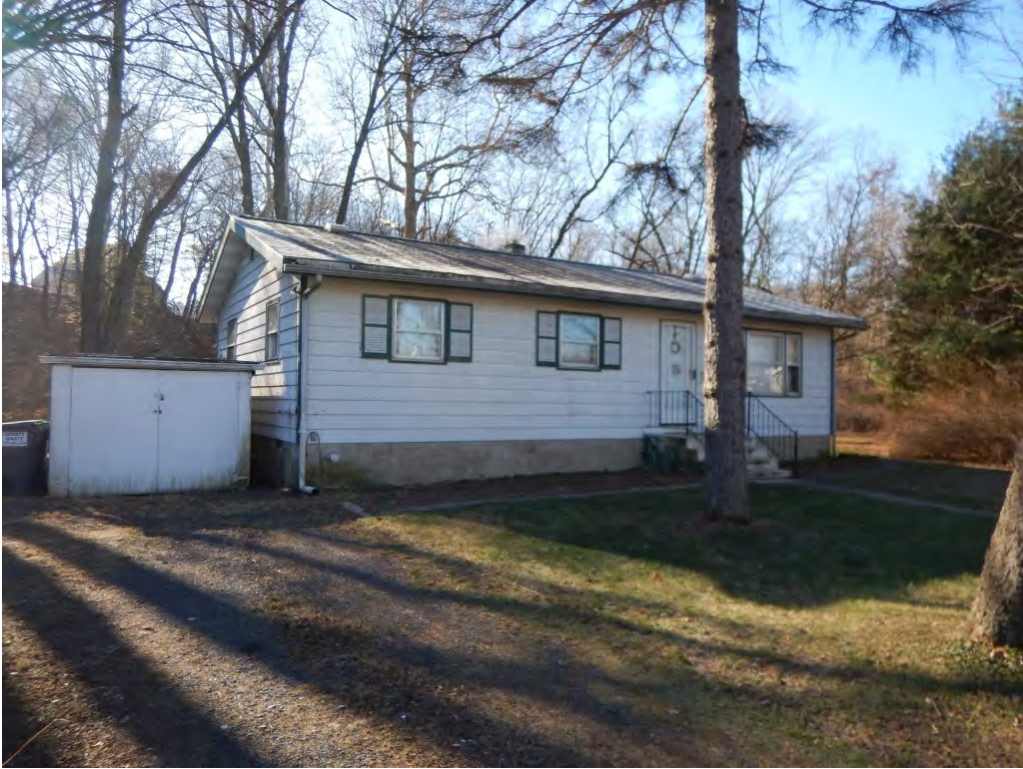
Photograph 9: View looking southwest at the north and east elevations of the house at 135 King David Road.
