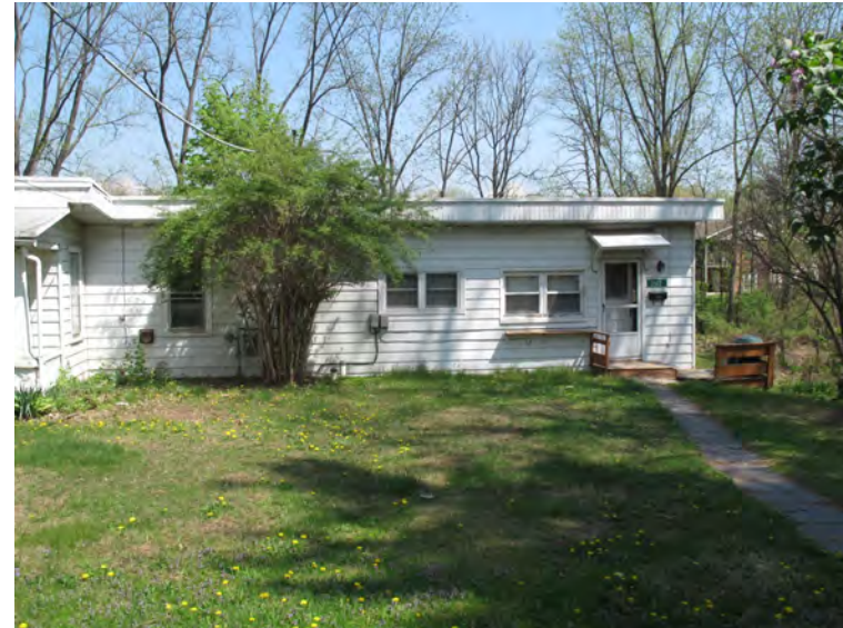
Caption: Photograph 1: View looking north at the south elevation of 3512 Pocono Park Drive.
