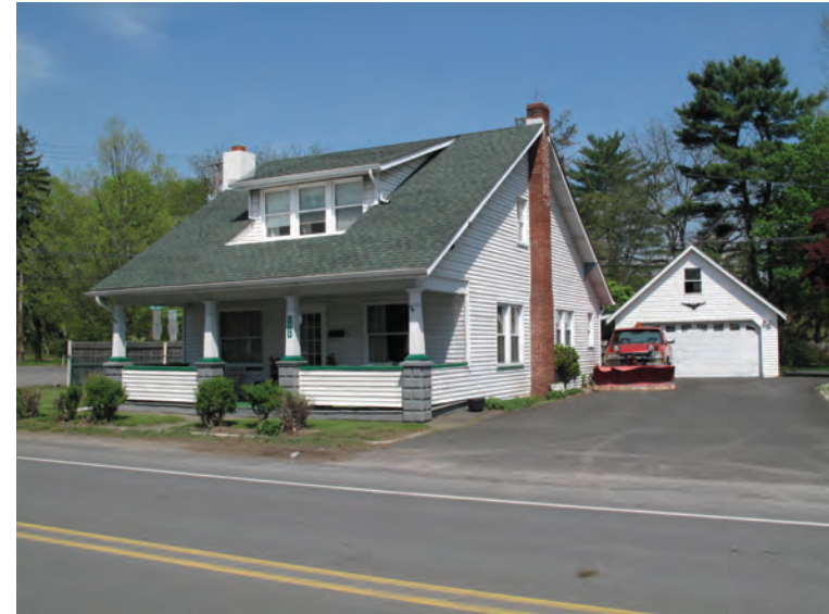
Caption: Photograph 1: View looking northwest at the south and east elevations of 1928 W. Main Street.
