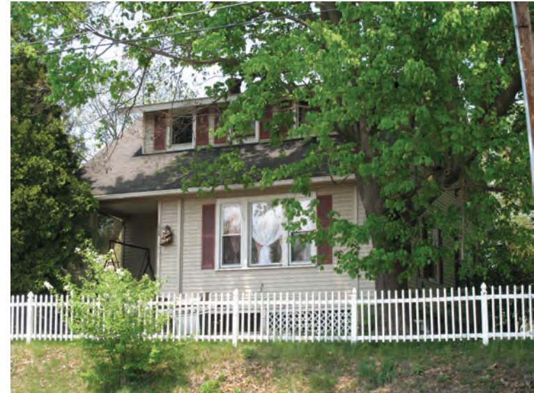
Caption: Photograph 1: South and west elevations of 1220 Dreher Avenue facing northeast.
