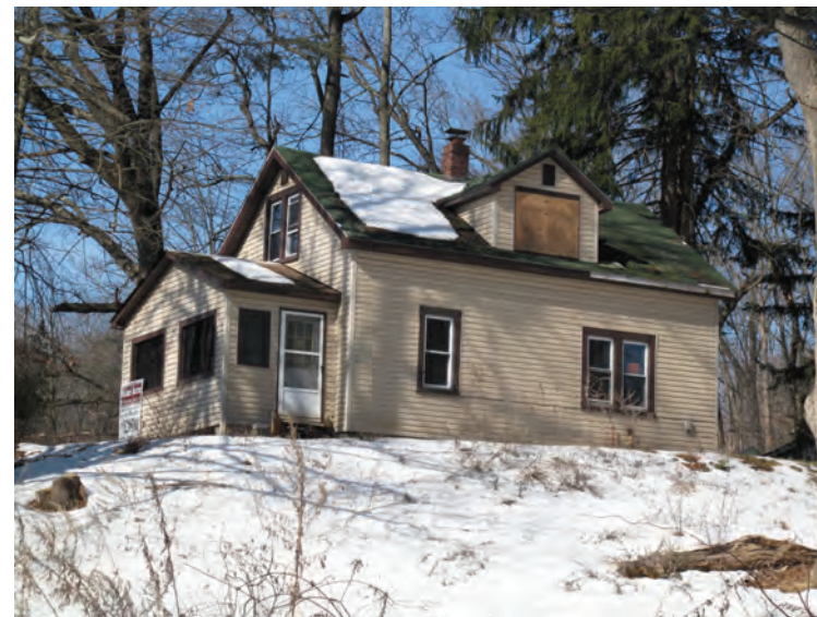
Caption: Photograph 1: North and west elevations of 353 White Stone Corner Road while facing southeast.
