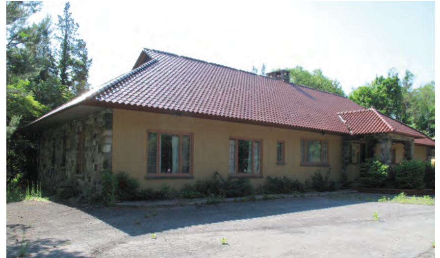
Caption: Photograph 1: View looking southeast at the north and west elevations of the Mediterranean style house at 1409 N. 9th Street.
