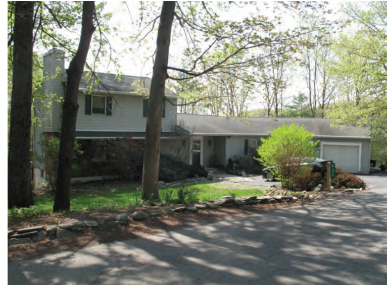
Caption: Photograph 1: West and north elevations of 433 Dogwood Road facing southeast.
