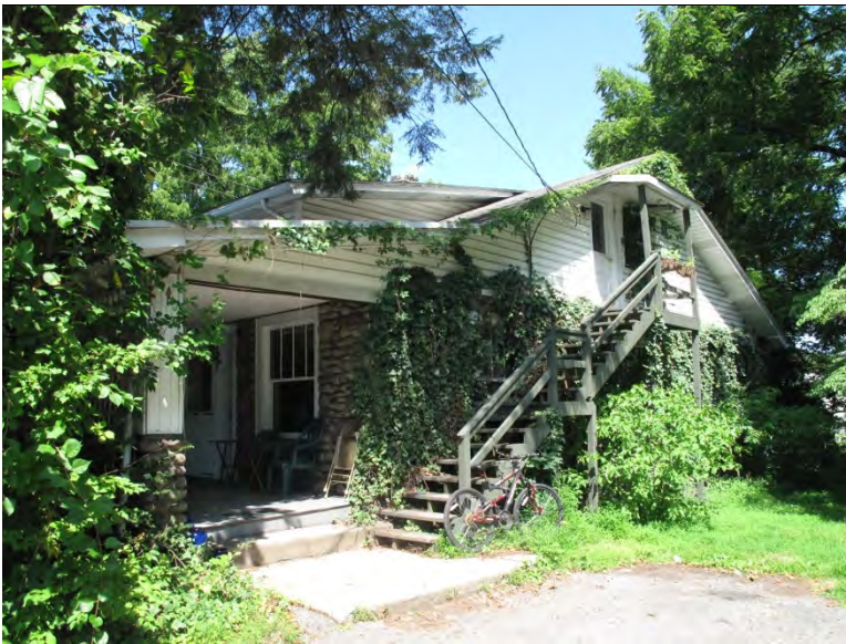
Photograph 43: View looking northwest at the east and south elevations of the Mengle House.
