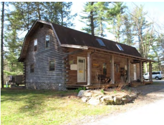
Photograph 34: View looking southwest at the north and east elevations of the Camp Office.
