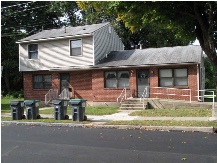
Photograph 4: View looking southwest at the house at 21/23 Garden Street.
