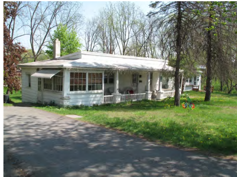
Caption: Photograph 2: View looking northeast at the south and west elevations of 3512 Pocono Park Drive.
