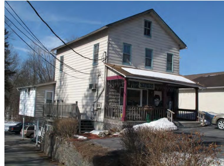
Caption: Photograph 1: View looking northwest at the south and east elevations of 1413 N. 9th Street.
