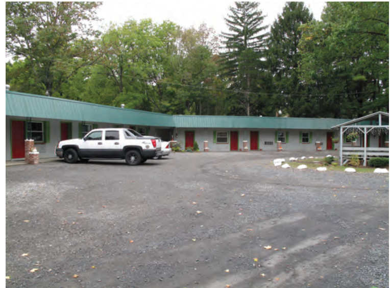
Caption: Photograph 2: View looking southwest at the L-shaped at the Flower Field Inn motel building at 1987 West Main Street.
