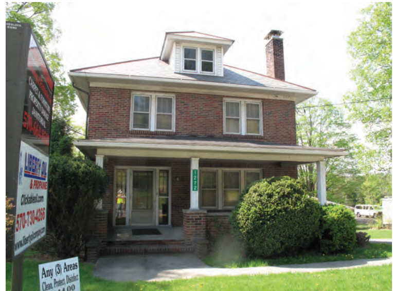
Caption: Photograph 2: View looking south at the north elevation of the Foursquare style building at 1272 N. 9th Street.
