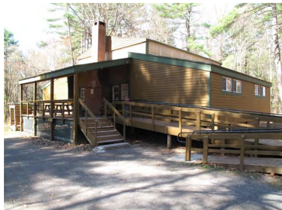
Photograph 35: View looking southwest at the north and east elevations of the Stroup House.
