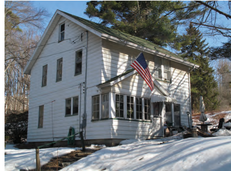
Caption: Photograph 1: View looking northeast at south and west elevations.
