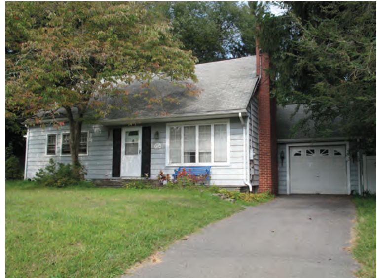
Caption: Photograph 2: South and east elevation of 1224 Dreher Avenue while facing northwest. The house is a modified Cape Cod style residence.
