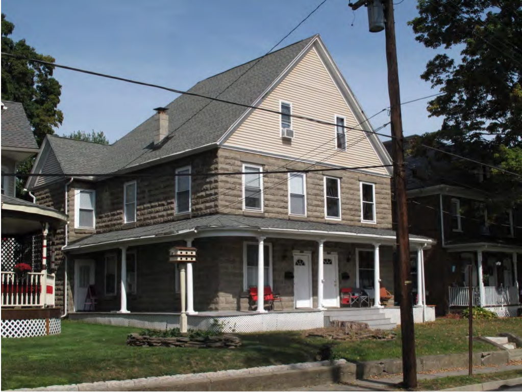
Photograph 3: View looking north at the south and west elevations of the house at 1080/1082 Dreher Avenue.
