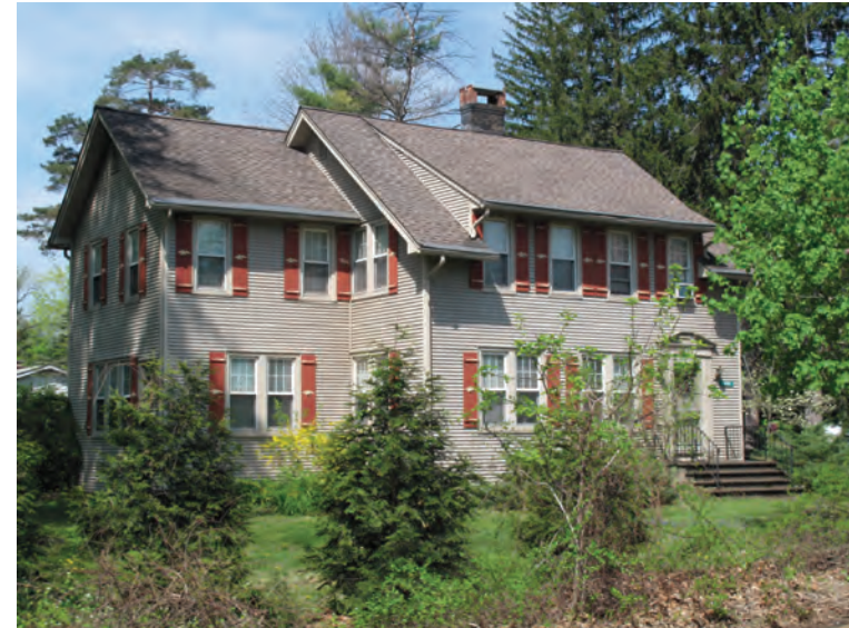
Caption: Photograph 1: View looking northwest at the south and east elevations of 3609 Bridge Street.
