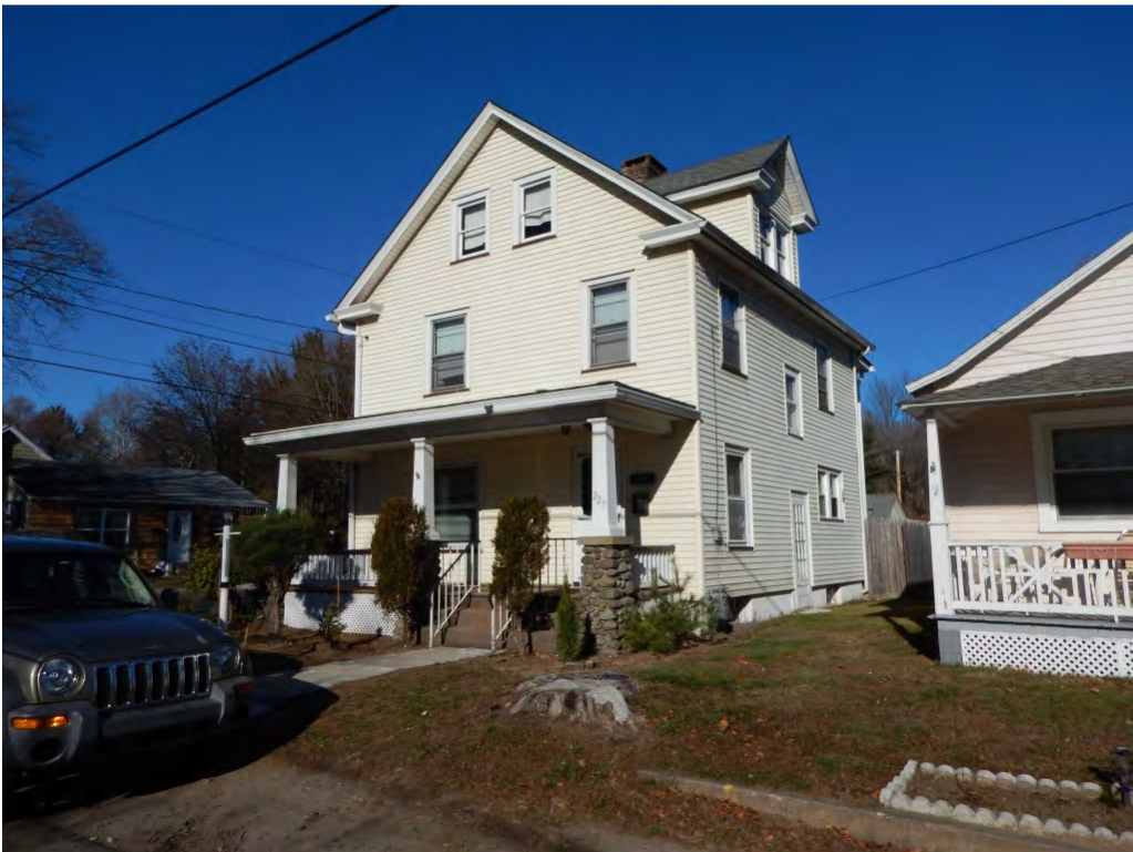
Photograph 6: View looking northwest at the east and south elevations of the house at 227 Pokona Avenue.
