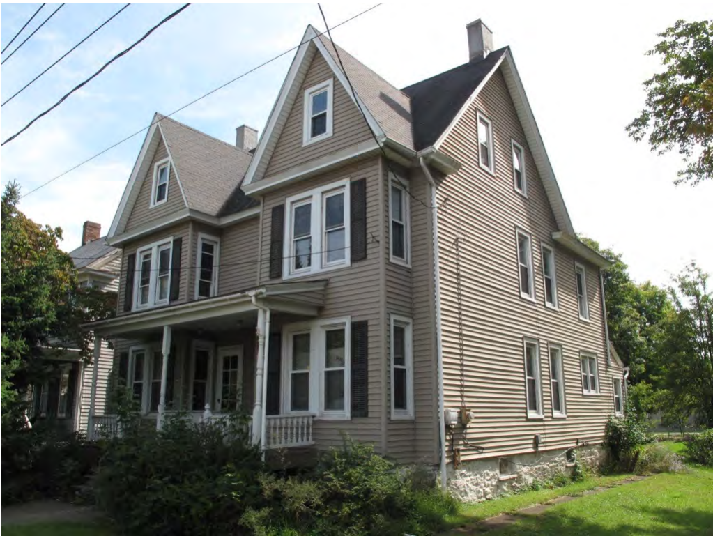
Photograph 4: View looking southeast at the north and west elevations of the house at 1053 Dreher Avenue.
