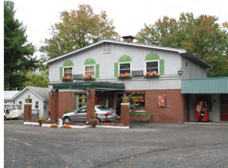
Caption: Photograph 1: View looking south at the north elevation of the Flower Field Inn office building at 1987 West Main Street.
