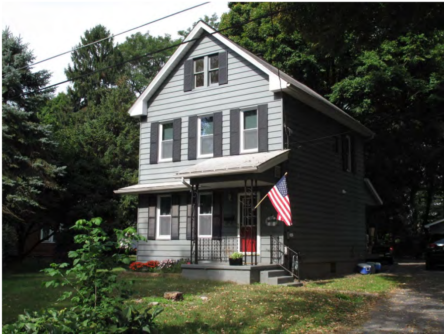
Photograph 4: View looking northwest at the house at 1131 Greenway Avenue.
