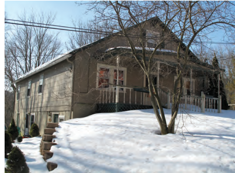
Caption: Photograph 1: North and east elevations of 315 White Stone Corner Road while facing southwest.
