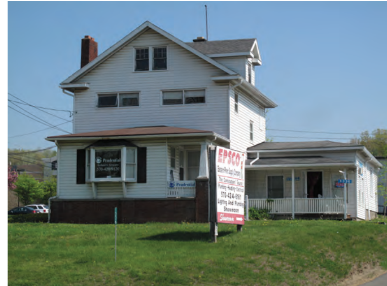
Caption: Photograph 1: View looking north at the south and east elevations of 1336 N. 9th Street.
