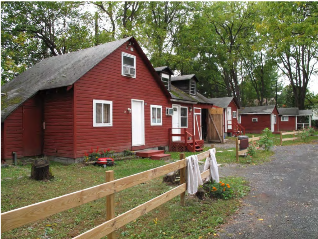
Photograph 4: View looking northwest at the cottages along the western edge of the Flower Field Inn property at 1987 West Main Street.
