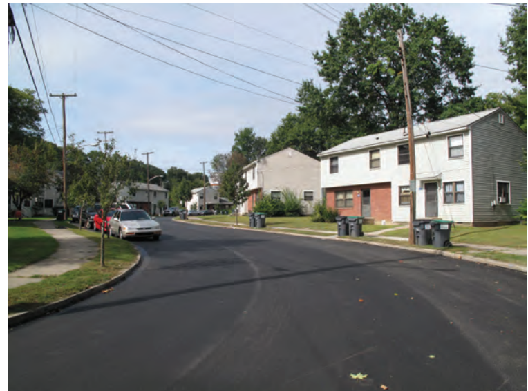
Caption: Photograph 2: View looking southwest along Garden Street at apartments 34/36 and 30/32 Garden Street.
