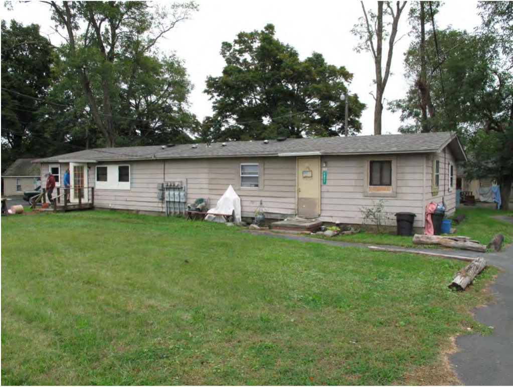
Photograph 5: View looking southeast at the building at 1971 West Main Street.
