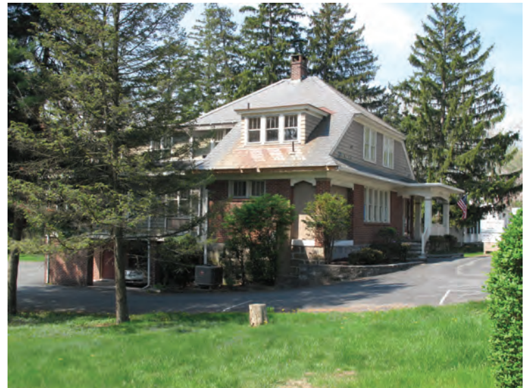
Caption: Photograph 2: View looking southwest at the north and east elevations of 1286 N. 9th Street.
