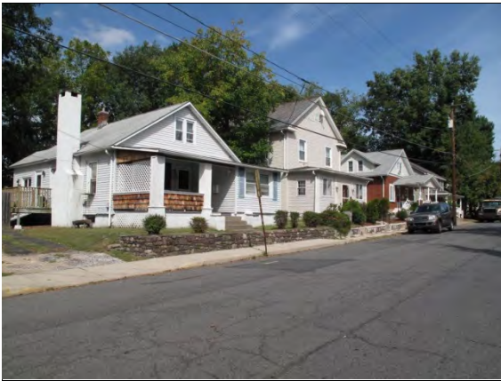
Photograph 40: View looking northeast along Lenox Street from Park Avenue.
