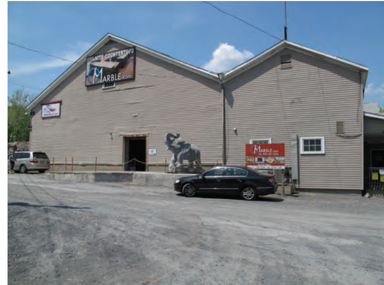
Caption: Photograph 1: View looking northwest at 65 Storm Street.
