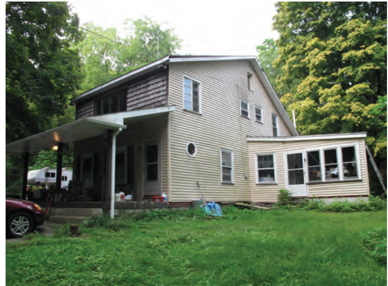
Caption: Photo 2: North and east elevations of 300 Tanite Road while facing southwest.
