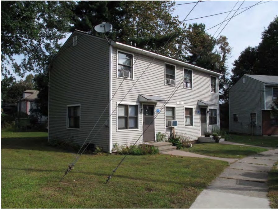
Photograph 3: View looking northeast at the house at 40/42 Garden Street.
