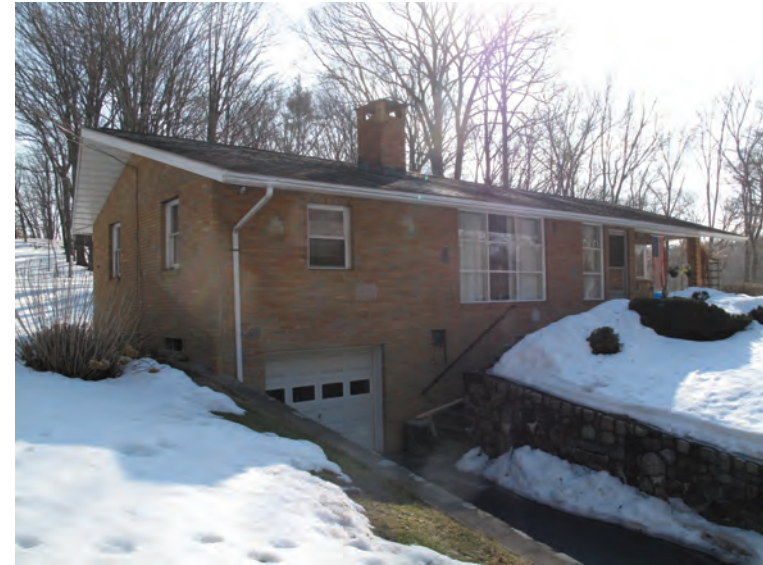
Caption: Photograph 1: View looking southeast at north and west elevations.
