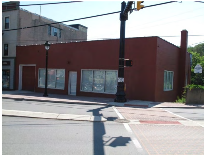
Photograph 49: View looking east at the north and west elevations of the Stroudsburg Motor Supply Company building.
