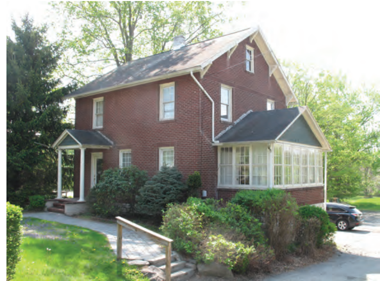
Caption: Photograph 1: North and west elevations of 1274 N. 9th Street facing southeast.
