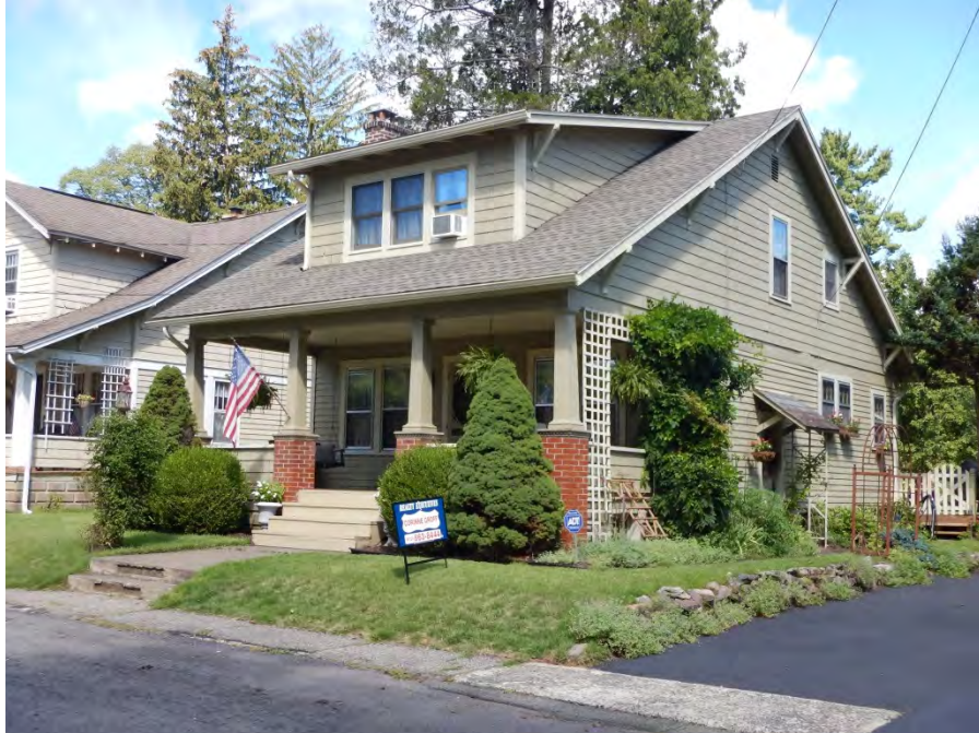
Photograph 5: View looking northwest at the south and east elevations of the house at 2030 Miller Street.
