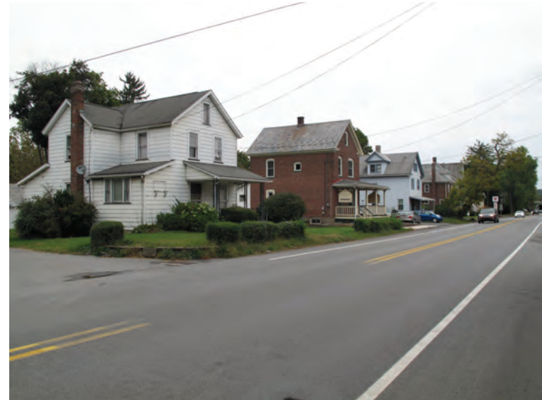
Caption: Photograph 1: View looking east along West Main Street from the intersection with Leafy Greene Street.
