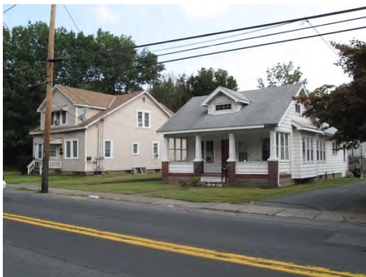
Photograph 22: View of residences located in the Bridge-Miller Street Grouping.
