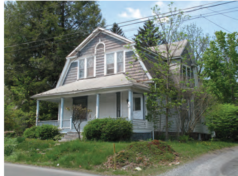
Caption: Photograph 1: View looking northwest at south and east elevations of 1222 Dreher Avenue.
