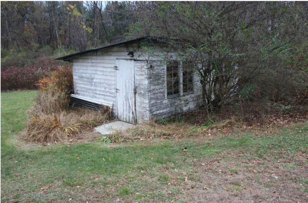
Photograph 6: General view of outbuilding associated with the house along White Stone Corner Road north of I-80, facing southeast.
