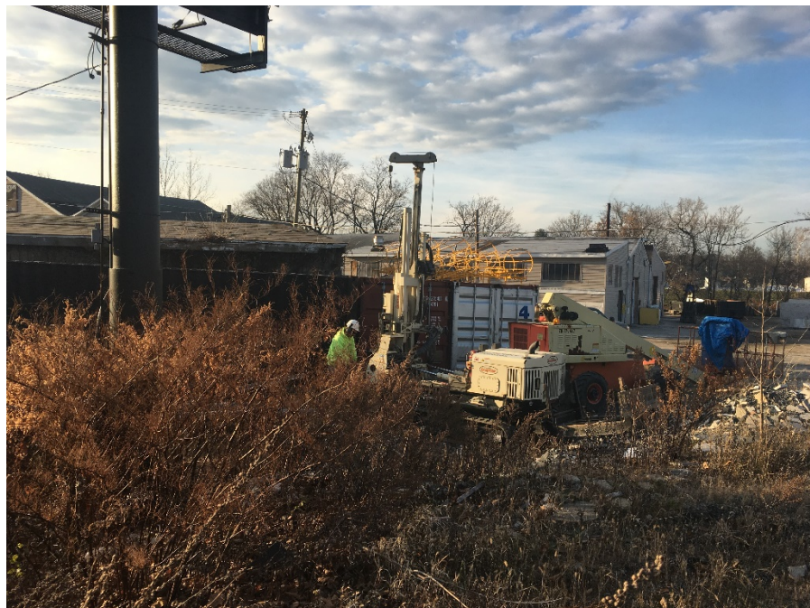
Former Research Laboratory site: geoprobe rig being set up.
