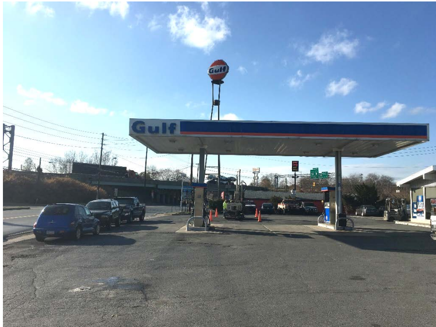
Pocono Gas Station site: geoprobe rig being set up.
