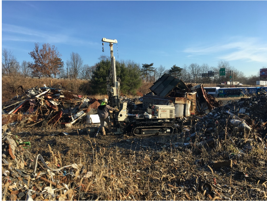
APS Recycling site: geoprobe rig set up to drill APS-GP09.
