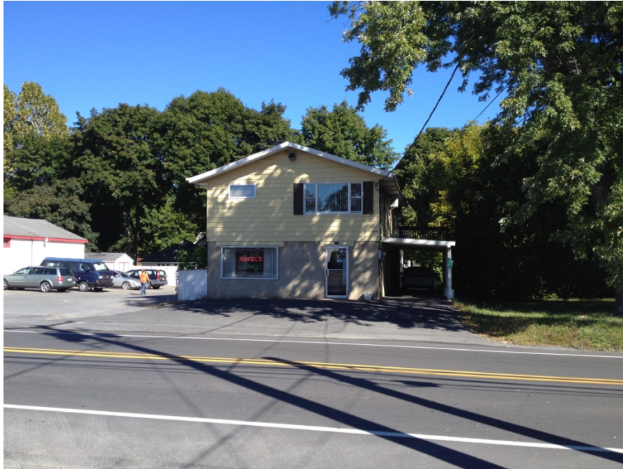
Klingel Cleaners and West Main Street PCE sites: view to the north.
