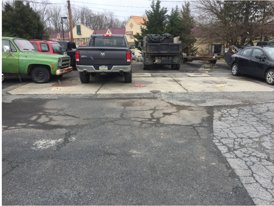
Pocono Gas Station site: view of existing UST field.
