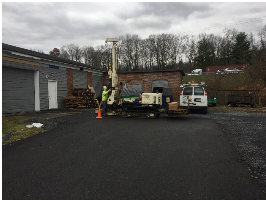
Perfection Shoe Machinery Company site: Geoprobe getting set up.
