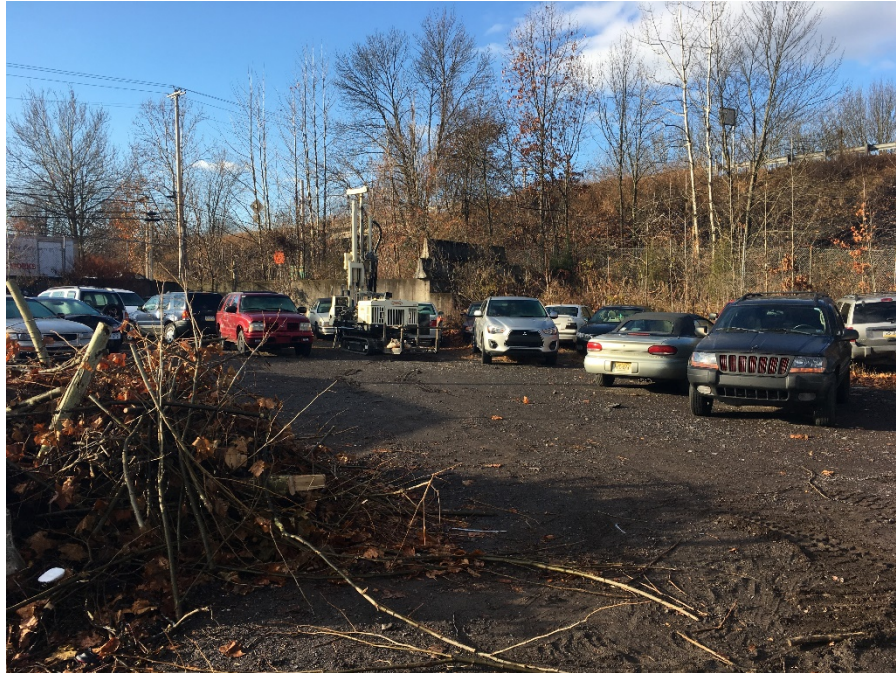
Rinehart EM, Inc. site: geoprobe rig being set up.
