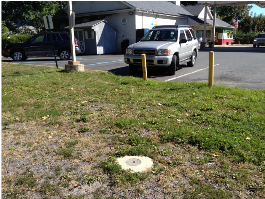
Main Street Stop and Go site: Monitoring well observed onsite, view to the northeast.
