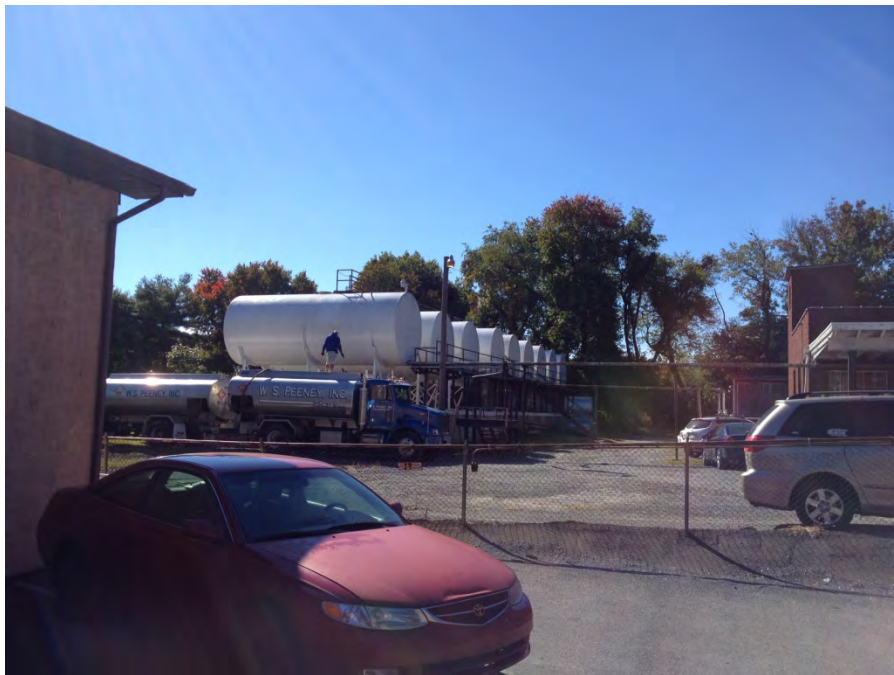
WS Peeney site from parking lot, view to the southeast.
