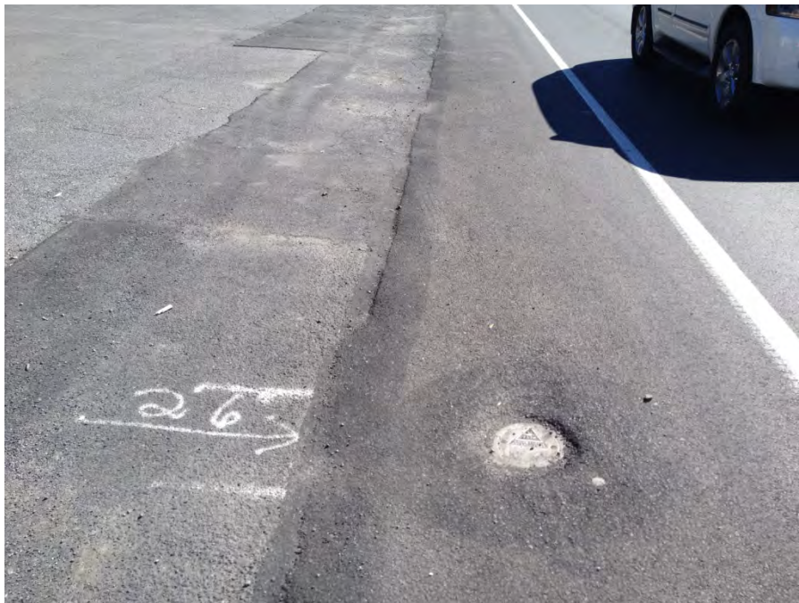
Monitor well observed in Main Street right of way in front of Klingel Cleaners, view to the east.
