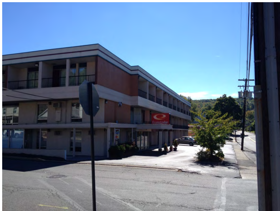
Former Total Auto Service site, view to the southeast.
