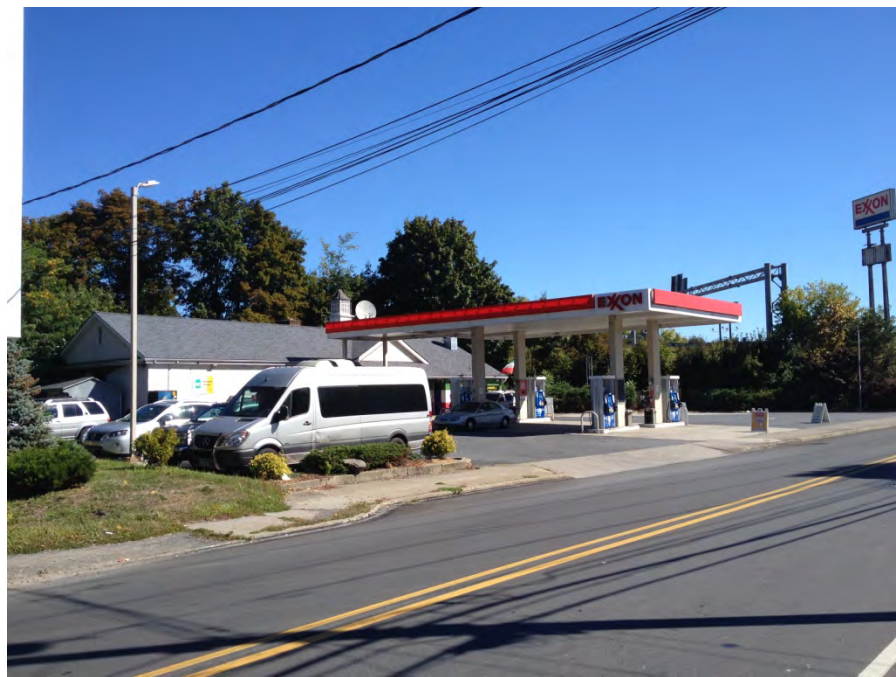
Main Street Stop and Go site, view to the northeast.
