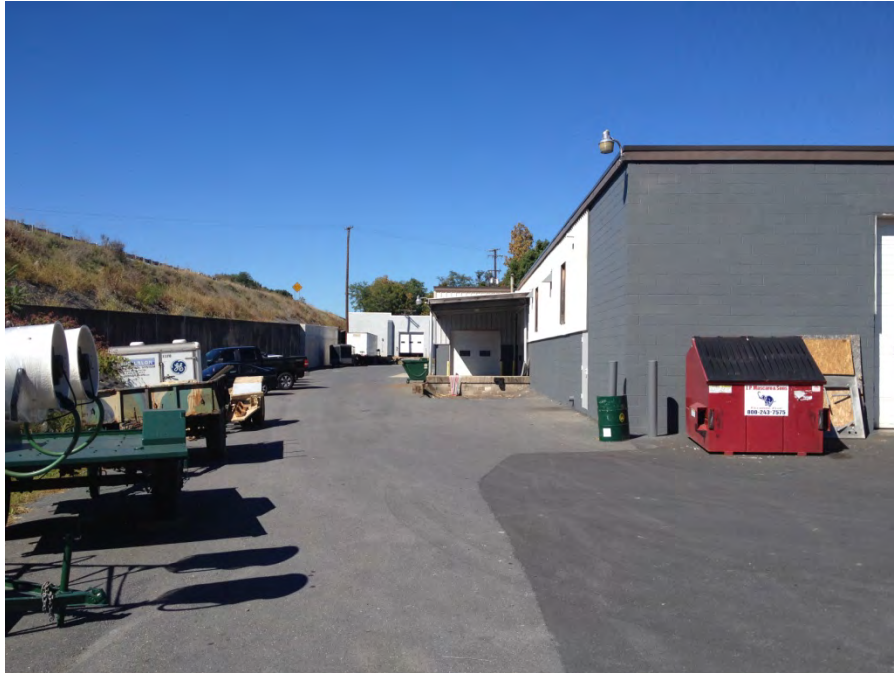
Biobuffer Solutions, Inc. site located within Pocono Foundry Site, view to the west.
