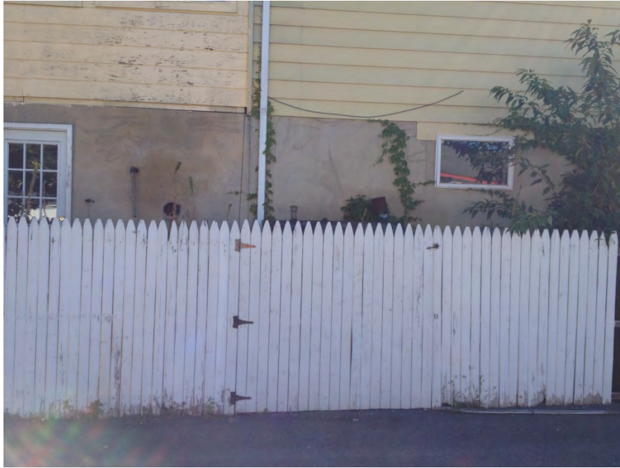
Heating oil AST observed adjacent to Klingel Cleaners building, view to the east.
